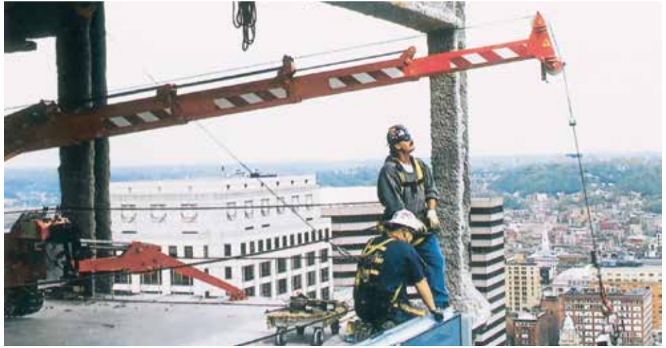
OPERATING ENGINEERS have no fear of heights as this member stands on the 34th floor of a building preparing to set windows.
