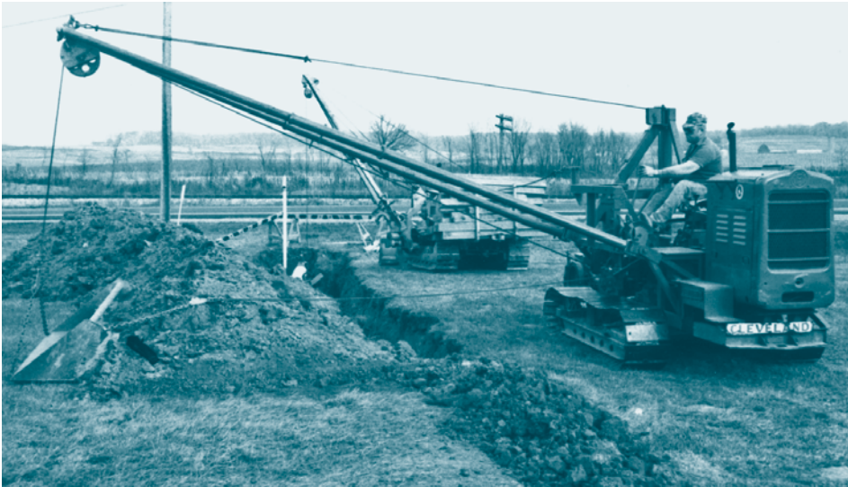
CLEVELAND drag box in use in the '50s, allowed operators to work safely when laying pipes.
