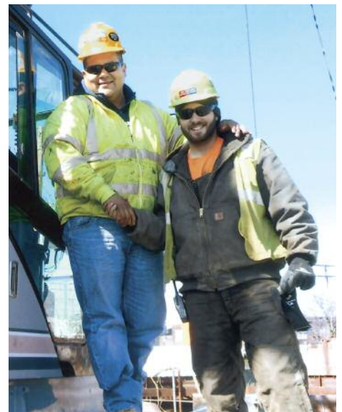
WORKING FOR Triad Engineering at the Dugway tunnel shaft #2 are (l-r) Jose Trewin (D-6) and Anthony Earhart.
