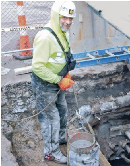
WORKING for Cook Paving on the CPP vault reconstruction is operator/helper Frank Simko.
