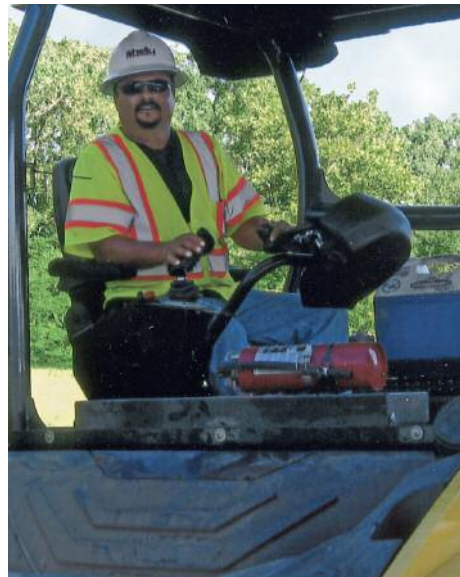
RUNNING an asphalt roller for Shelly on S.R. 15 is Rick Gardner.
