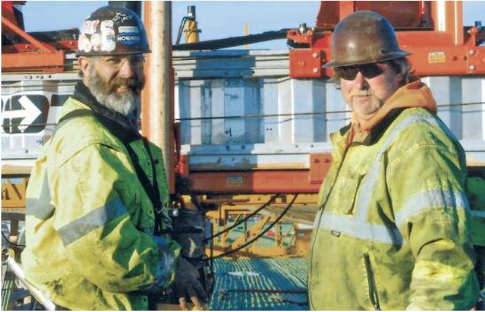
OPERATING a pump truck for Howard Concrete Pumping on the I-90 Innerbelt Bridge are (l-r) Bob Husted and William Meier.
