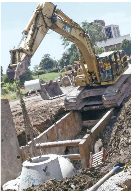
SETTING 72" concrete pipe on the Black River tunnel for Ric-Man Construction is John Burrington.
