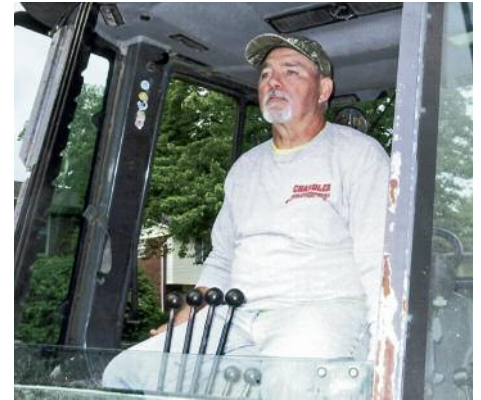
WORKING on a curb and sidewalk replacement is Bill Kidd, on the job for R.A. Miller.
