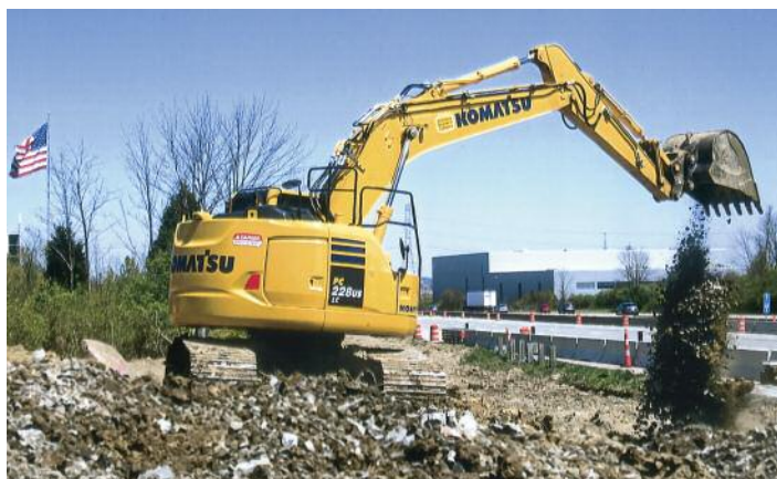
REPLACING bridge at Socialville Foster Rd. and I-71 for Eagle Bridge is Doug Nagel.
