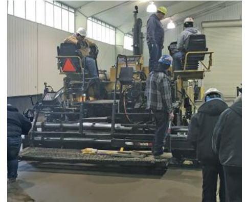
ASPHALT PAVING in an all-weather building at the Logan training site.
