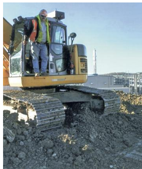
HANDLING site work for Kokosing at the MarkWest Seneca processing plant is Ralph Dalton (D-3).
