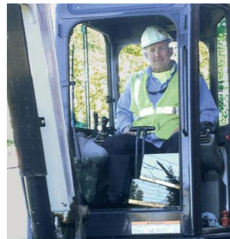
WORKING at the Heatherdowns pump station in Toledo is Robert Draper, owner-operator of Draper Excavating.
