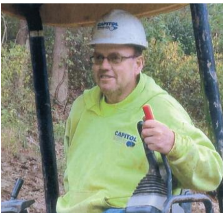
S.R. 7 in Chesapeake has Mark Pennington on the job for Capitol Tunneling.
