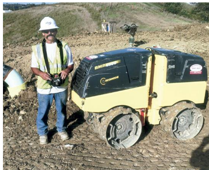
WORKING on Otis Eastern hot taps for Spectra Energy is James Snyder.
