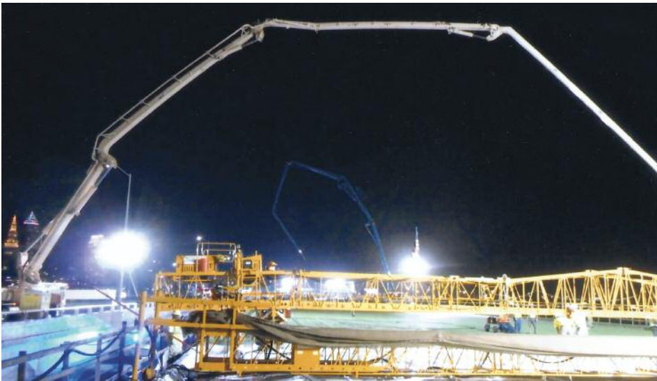
PUMPING concrete by Howard Concrete Pumping at the final pour on Cleveland's Innerbelt Bridge.
