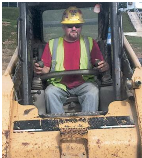
FOOTBALL Hall of Fame project is keeping Eric Johnson (above) busy for Beaver Excavating and Rick Ross and Bob Jarvis (l-r right) busy for Canton Erectors.
