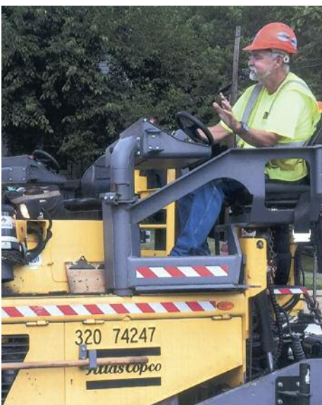
RUNNING a paver is Alex Farren, working for Central Allied in Canton.
