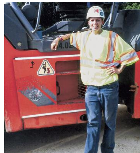
WORKING on Shelly's turnpike project in Portage County is Jennifer Miller.
