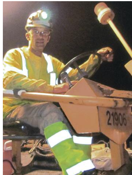
WORKING on the I-271 road widening is Grant Massey II working for Kokosing.
