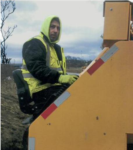
OWNER OPERATOR Randy Dotson (D-1) working on I-271/I-77 lighting for Zenith Systems.
