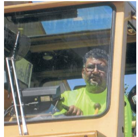
S.R. 65 slide repair is being handled by Herman Kennedy (D-3) for Shelly & Sands.
