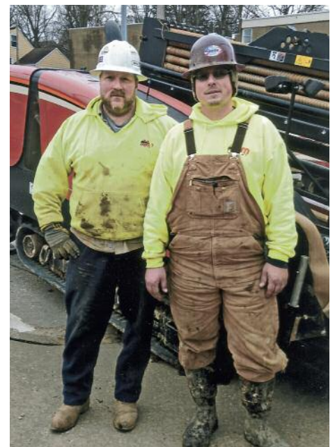
RELOCATING gas lines on Summit St. in Kent for H.M. Miller are (l-r) David Snure and John Shircliff.
