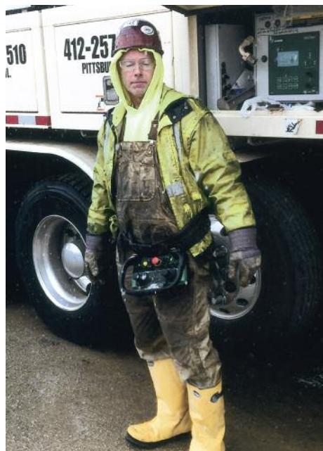
PUMPING concrete for Howard Concrete Pumping on the Ledge Rd. bridge foundation is Ed Vanko.
