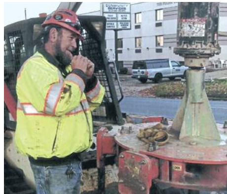
RUNNING a skid steer with a manhole saw attachment is Marty Brumbaugh working for Northstar.
