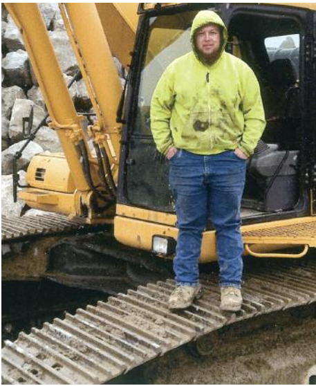
STACKING armor rock in Fairport Harbor for Huffman Equipment is Jeremiah Klingman.
