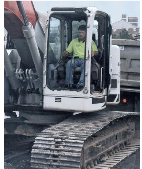
REHAB of Morrison Rd. in Toledo is keeping Brian Yeager busy for Crestline Paving.
