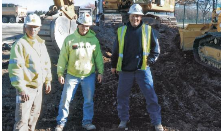
DOING site work for Platform Cement at Burke Lakefront Airport are (l-r) Mike Lauria, Tom Cooper and Dave Castilyn.
