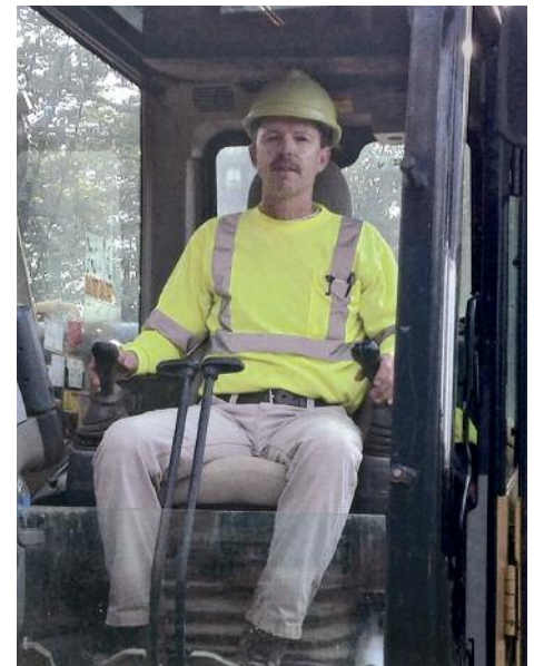
WORKING on a Thorpe Rd. bridge rehab in Berlin Heights is Donnie Saalman on the job for Schalk Brothers.
