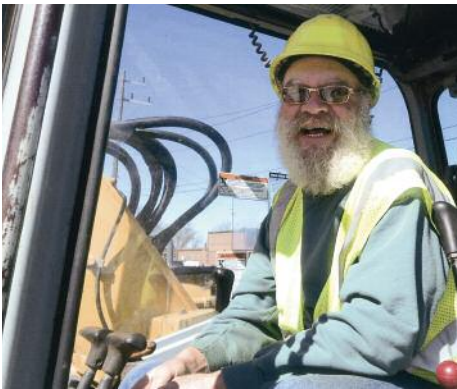
WATER LINE work has Norm Olszewski (above) working for Terrace Construction and Chris Williams (right) on the job for Fabrizi.
