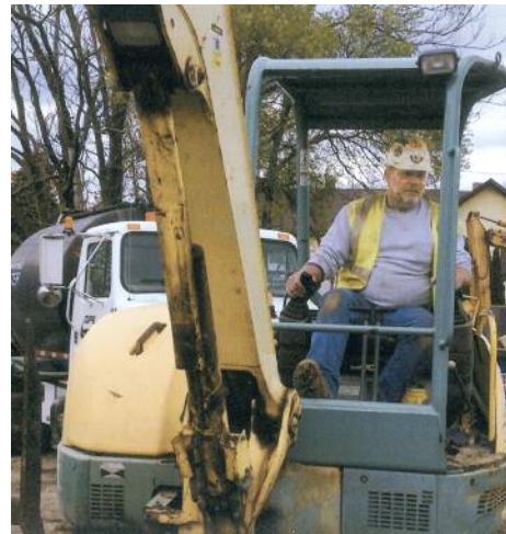
NEW Local 18 contractor F.E.T. Contractor Services has John Longberry working on the Anthony Wayne Trail.
