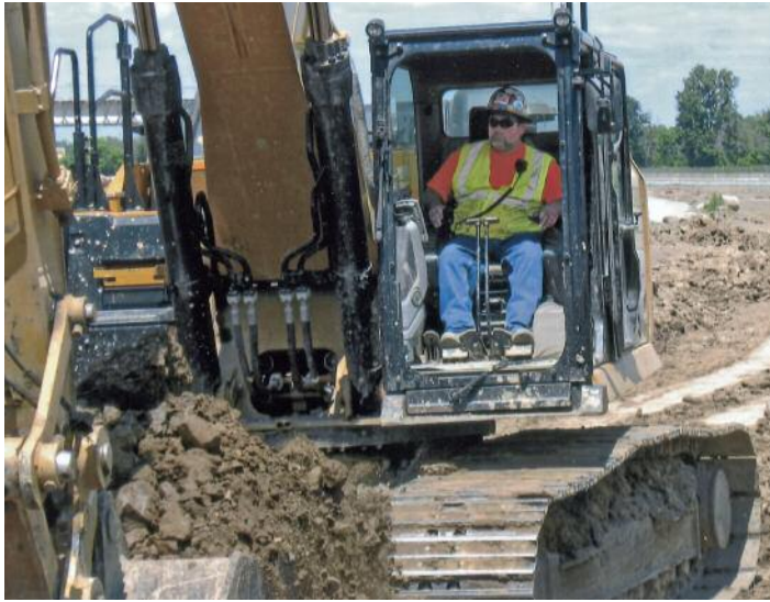
WORKING on Beaver Excavating's I-75 reconstruction in Lima is Rob Fisher.
