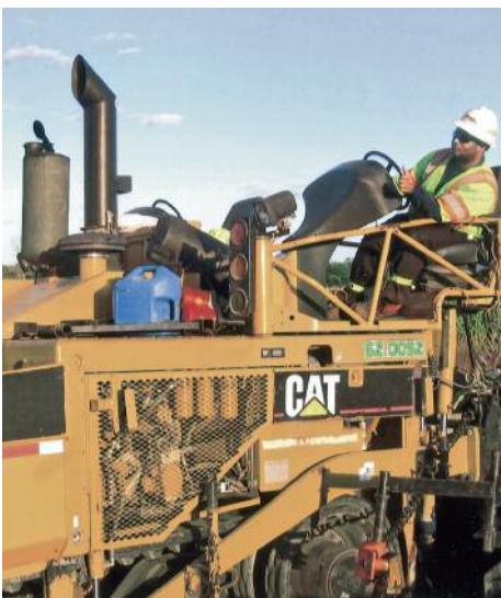
WOOD COUNTY projects have James H. James (top) and Mike Higgins (above) working for Shelly on I-75, and Brian Kolodziejczk (right) on a paver for Gerken Paving.
