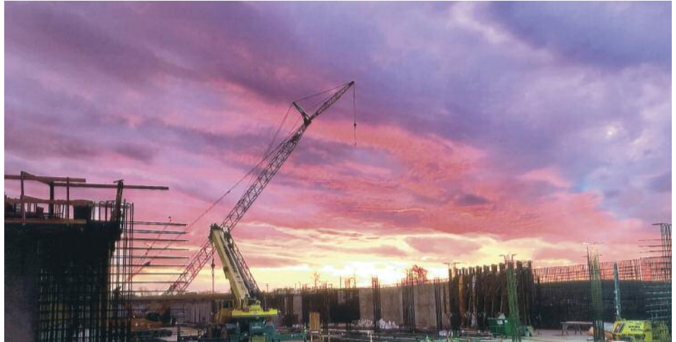
SUNRISE over Kokosing's Parsons Ave. water treatment expansion in Columbus.
