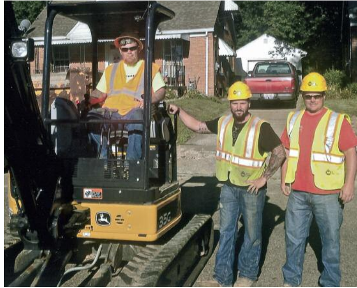
GAS MAIN work is being handled by Russ Miller (D-1), Mike Nestor and Matt Miller (left) for Miller Pipeline in Alliance. (Below) Luke Ruble is working in Navarre for KS Energy Services on a similar job.
