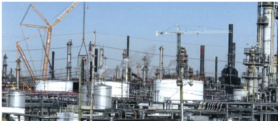
DAY & NIGHT work continues at the Husky Refinery as Deep South Crane & Rigging uses a 1,600 ton Terex PC 8800 Demag crawler crane.
