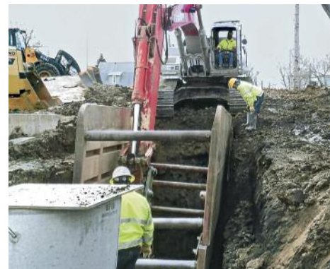
INSTALLING a 48-inch reinforced concrete storm pipe at Miller Brothers' CSO in Toledo is Doug Dennison.
