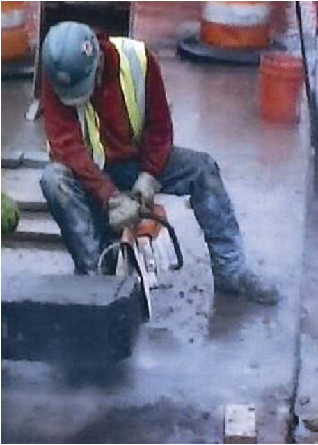
INSTALLING granite curb for Utilicon in downtown Cleveland, Dave Bigler is operating a two-cycle concrete saw.
