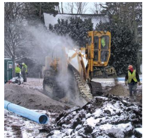
WORKING for Underground Utilities on a water line project in Portage is Mike Gerber .
