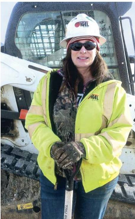
WORKING for George J. Igel at AEP's substation in Mt. Sterling is Tracy Powers.
