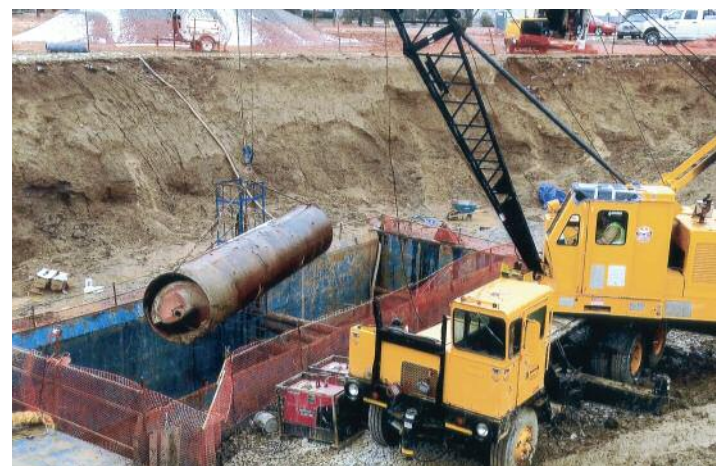
TURN-KEY TUNNELING in south Columbus.
