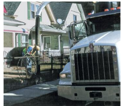
WORKING on a hydro excavation gas line replacement is Levi Crooks, on the job for Miller Pipeline (right).
