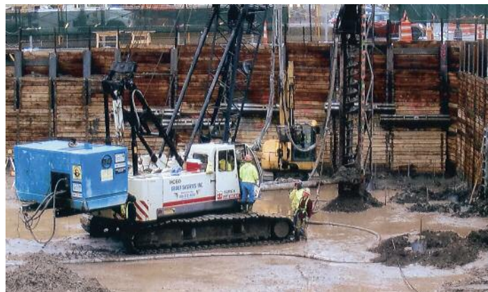
DRILLING auger cast piling, Grout Systems is working on a new office building for the city of Columbus.
