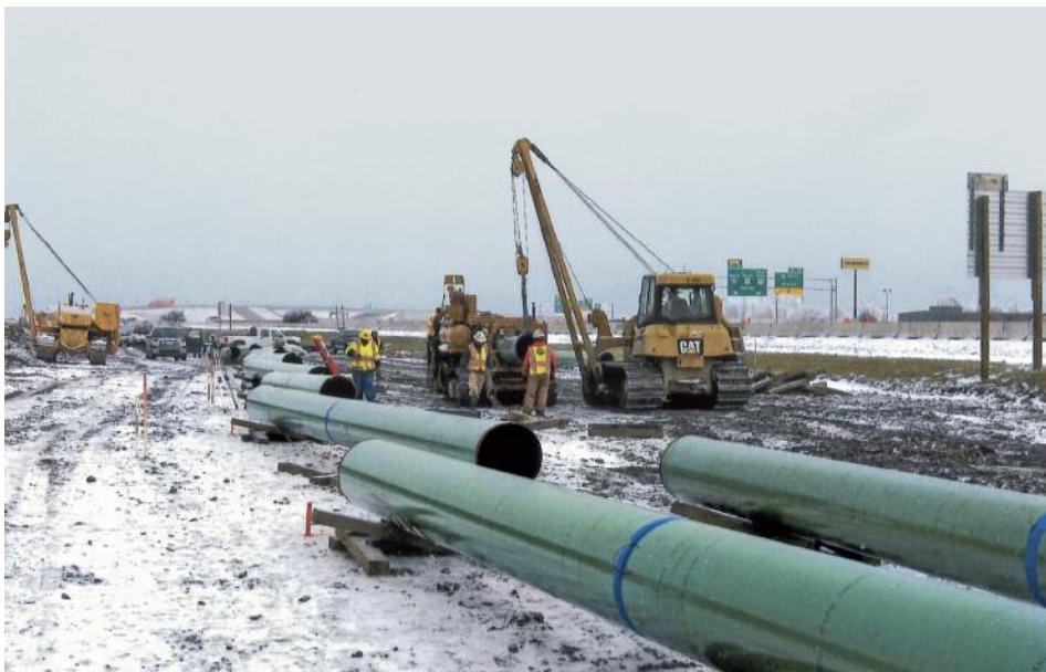
WELDED CONSTRUCTION bending crew working on North Coast gas transmission line on Oregon lateral line in Perrysburg.
