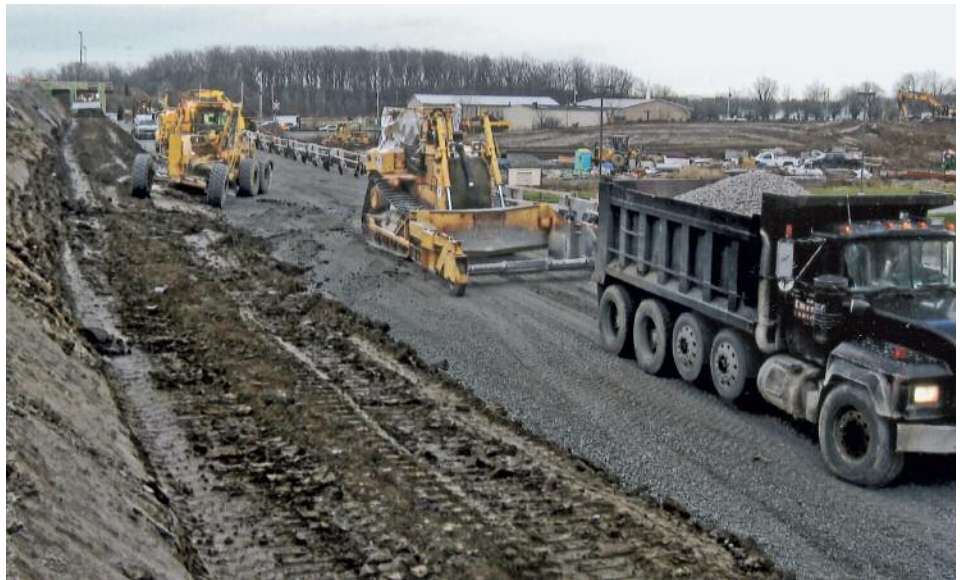
BEAVER EXCAVATING building an MSE wall on its I-75 reconstruction in Lima.
