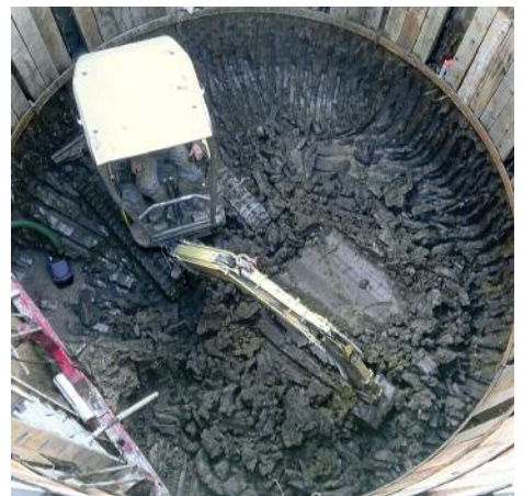
CHRIS HISER (above) working for HPH "clamming" with a 35-ton Grove Picker and (below) excavating using mini-clammer with picker in 42-foot shaft.
