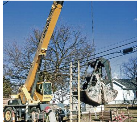
CHRIS HISER (above) working for HPH "clamming" with a 35-ton Grove Picker and (below) excavating using mini-clammer with picker in 42-foot shaft.
