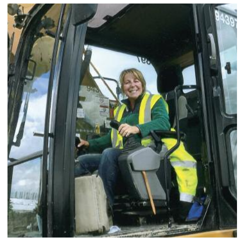
HANDLING a CAT 336 excavator on the I-75 reconstruction in Toledo is Angela Thourot working for Kokosing.
