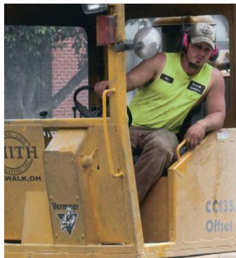
RUNNING a Vermeer saw for Smith Paving in Tiffin is Jim Roeder.
