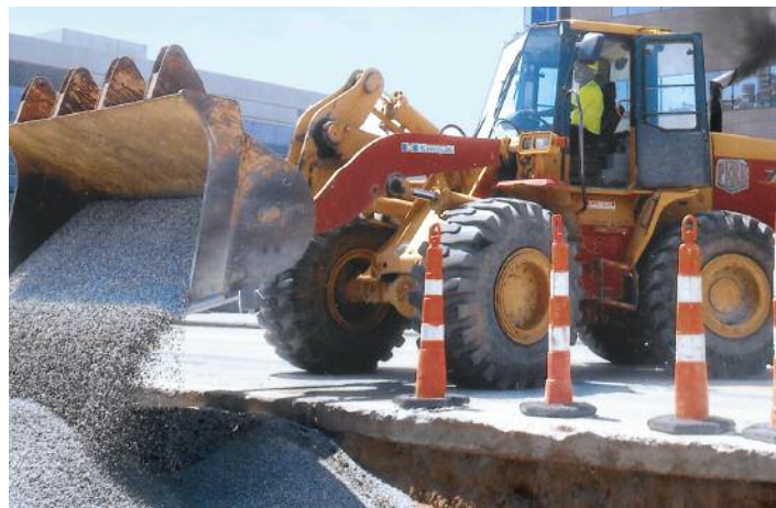
OPERATING a front end loader, James Bell is on the job for McTech on the Opportunity Corridor .
