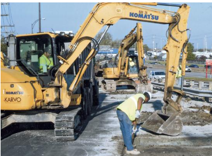
USING an excavator for joint repairs on S. Marginal Rd. in Cleveland is Dave Romano, working for Karvo Paving.
