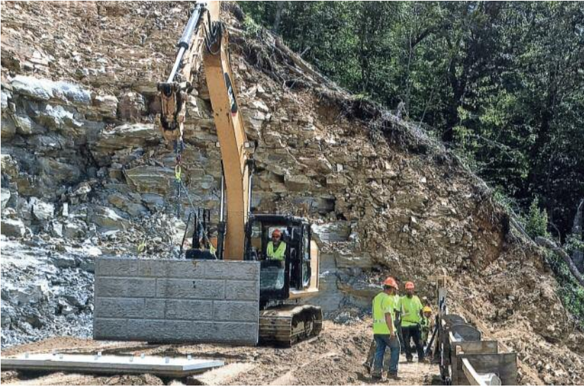
SETTING panels for a bridge abutment on the Portsmouth Bypass is Andy Fuller working for Beaver Excavating.
