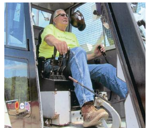
OPERATING a crane for Kelley Steel Erectors is Jim Reffner at Lakeland Community College.
