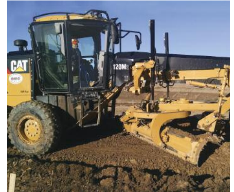
GRADER CLASS at Cygnets with Dave Gates cutting a road.
