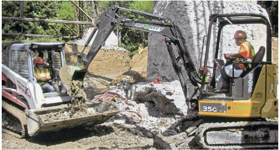
REPLACING piers for Norfolk Southern RR while working for Lane Construction in Ashtabula are (l-r) Devi Bagley and Reuben Lynch.
