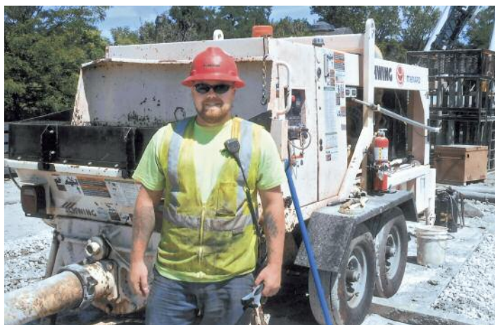
MANNING a Schwing concrete pump for Nicholson Construction is Ron Schoeppner (D-6) on shaft 4 of the Dugway storage tunnel.
