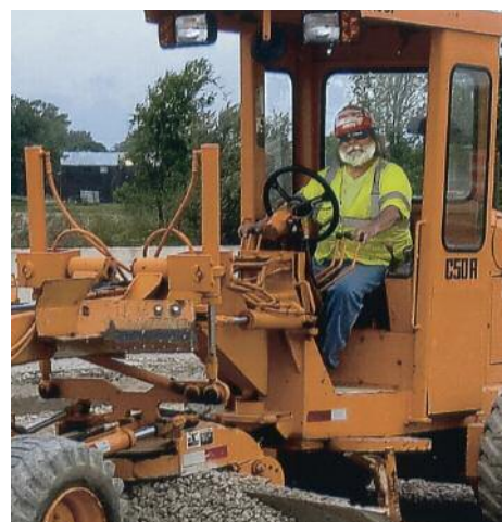
FINISH grading stone in Canal Winchester is Kendal Miller on the job for Kokosing.
