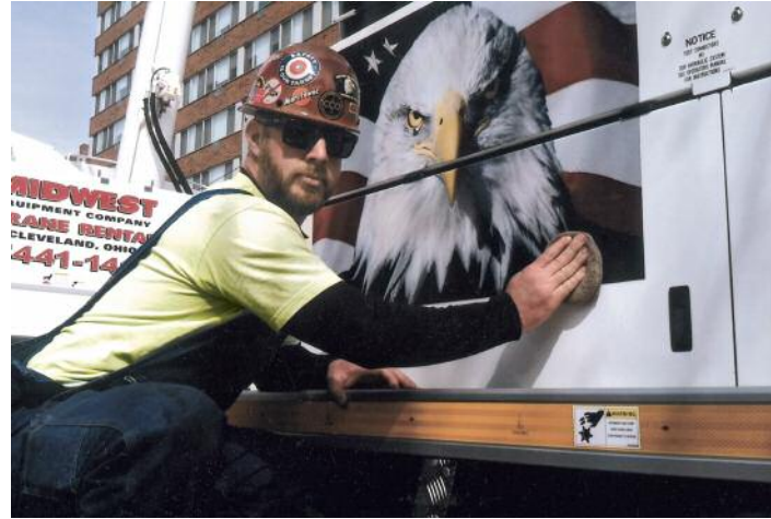
OILING for Dennis Hosler is Steve Rachkofski at the Barton Towers cell antenna in Lakewood, both working for Midwest Equipment.
