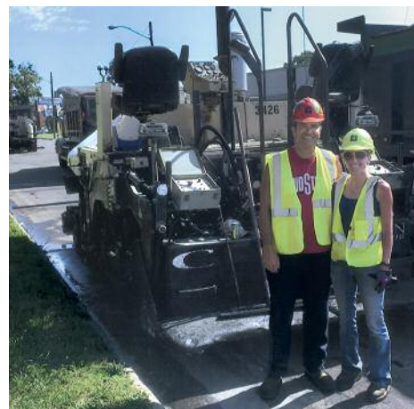
PAVING 12th St. in Canton are Jim and Danielle Carlisle, working for Central Allied.
