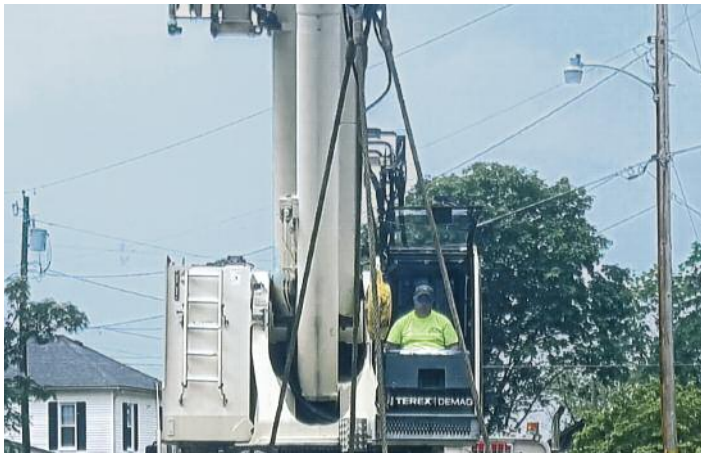
SETTING box culverts for Ohio-West Virginia Excavating in New Matamoras is Shane Nichols working for All Crane.
