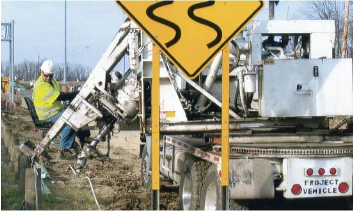
PULLING guardrail posts for Lake Erie Construction on I-270 is James Jenkins.
