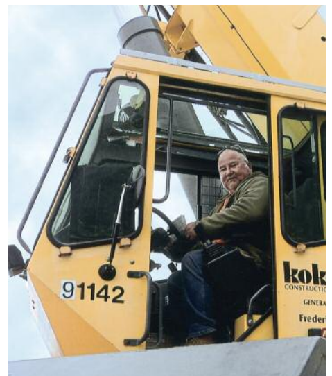
OPERATING a rough terrain crane, Patrick Rockett is working for Kokosing at the Southerly WWTP.
