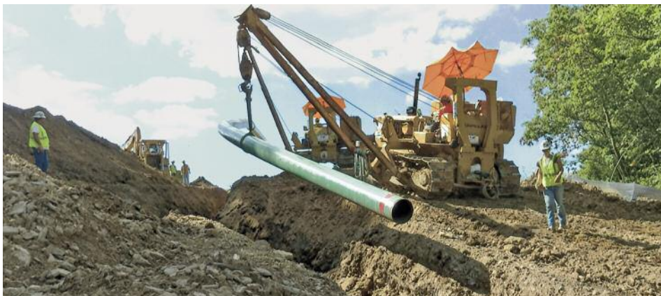
PIPELINE construction company Price Gregory working on its Marathon pipeline in Dover.
