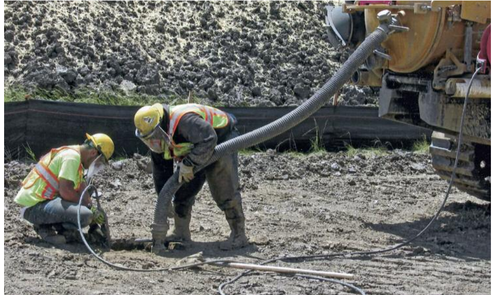
CONSTRUCTION of the Oregon Lateral Pipeline is keeping many D-2 members busy for Welded Construction. (Above) Mitchell Darrington, working with a laborer, mans a hose operating a pothole rig. (Below right) Ronnie Briscoe operates a John Henry rock drill as does Brianne Perez (below left).
