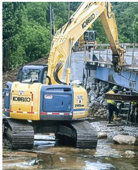
BRIDGE WORK on S.R. 150 in Jefferson County has David Tilley working for Shelly & Sands.
