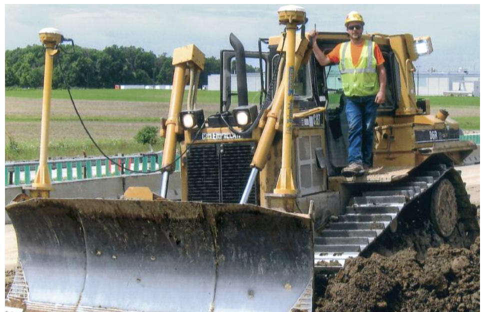
RUNNING a finish dozer on Beaver Excavating's I-75 reconstruction in Lima is Larry Lee (D-3).
