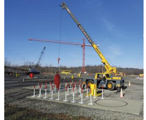
APPRENTICE GRADUATE Layla Hemsoth practices crane maneuvers at Richfield.
