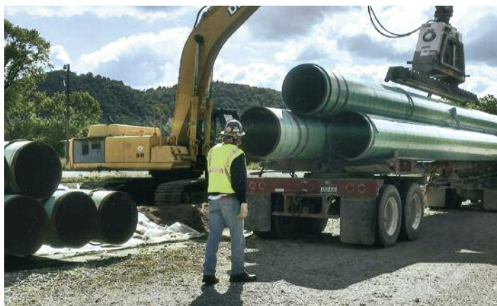
LOADING pipe for Ace Pipeline in Monroe County is Steve Hockenberry.
