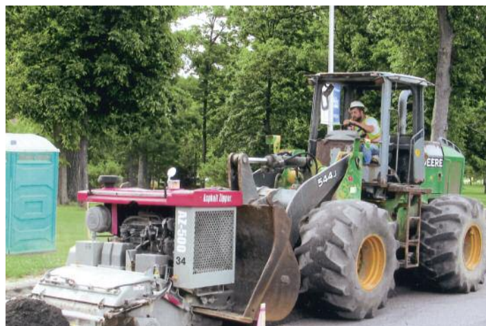
OPERATING a loader with an asphalt zipper attachment is Jarrid Miller, working for Helms & Sons.
