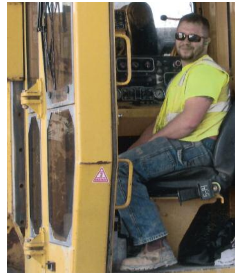
TRENCHING underdrains for Kokosing on I-75 in Wood County is Justin Lynch.
