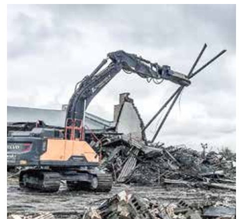
ON THE JOB in Newark, Licking County is Loewendick Demolition.
