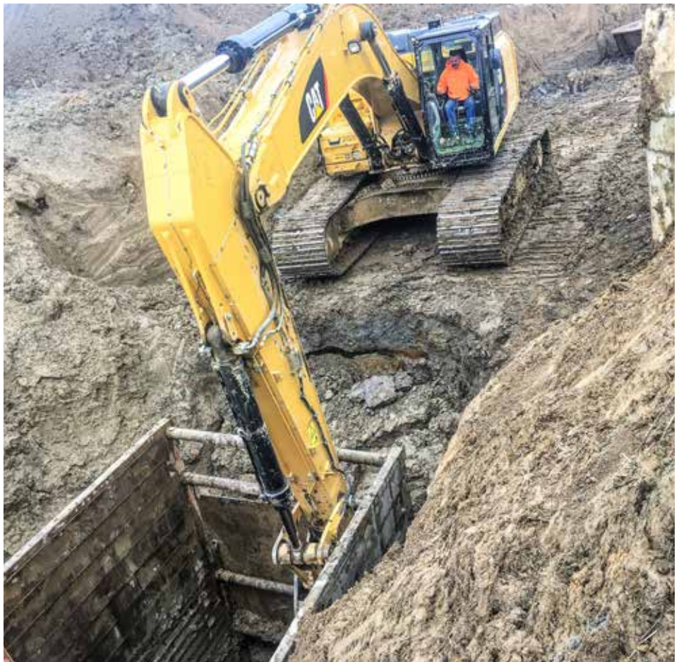
DIGGING for Fechko in Delaware County is Todd Armstrong.
