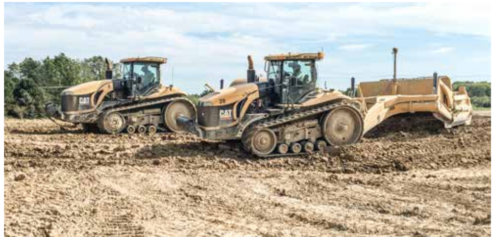
MOVING dirt for a subdivision on Hollstein Drive in Amherst is Kostecki Excavating. Tyler Fleck is operating the challenger pull pan on the left and Logan Fleck is operating the challenger pull pan on the right.
