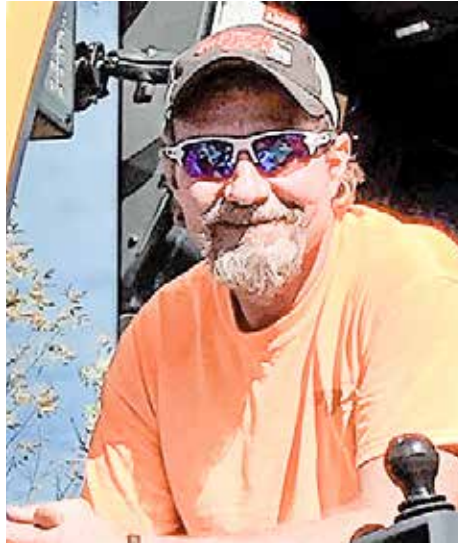
SETTING box culvert in Fairfield County for Capital City Crane is Brian Johnson.
