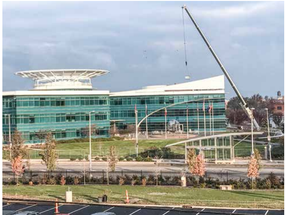
ALL Crane setting panels for Allied Corporation in Cleveland.
