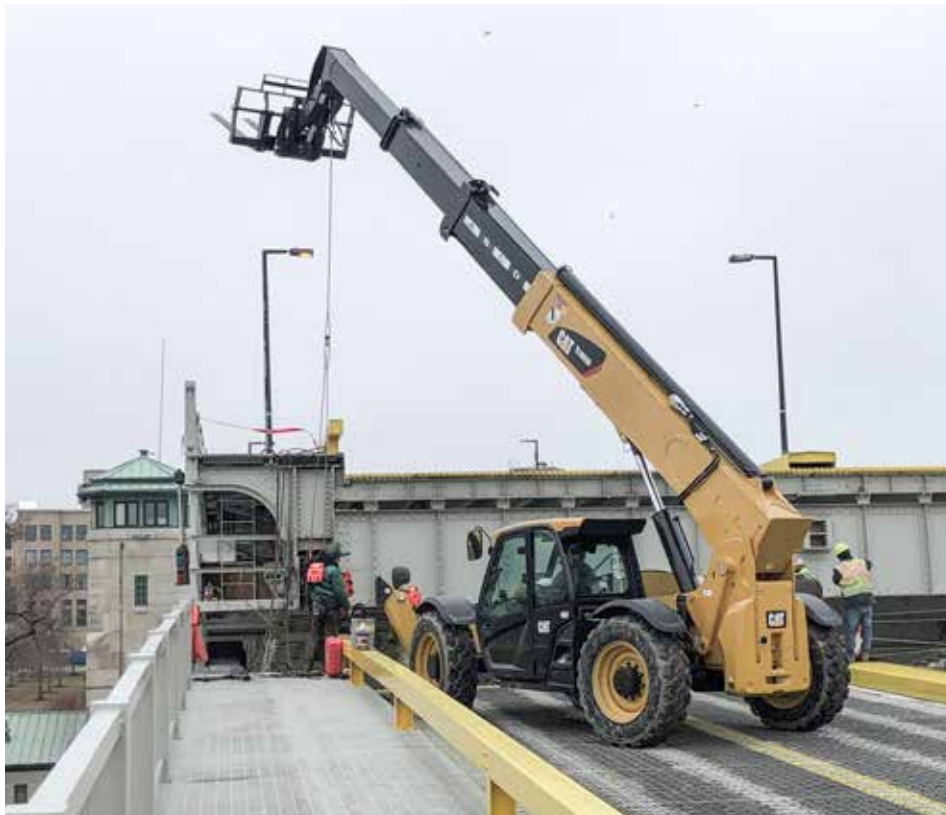
REPLACING the bridge locks on the Charles Berry Bridge in Lorain for Ruhlin is rough terrain forklift operator Matthew Veselko.
