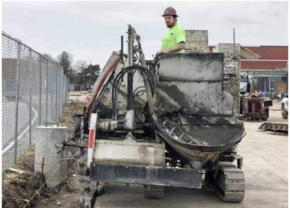
TRIMMING for a new curb at the new middle school in Sandusky for Smith Paving is Dave Brown.
