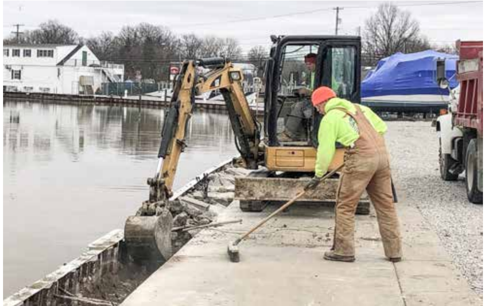
REPLACING the sheet piling with a mini excavator for Herk Excavating at the Vermilion Power Boats yard in Vermilion, is Dan Young.
