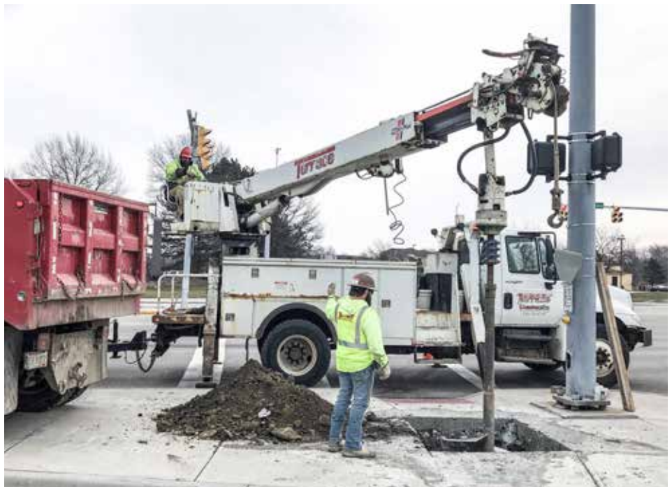
DRILLING foundations for new traffic light posts on S.R. 252 in North Olmsted for Terrace Construction is Phil Harter.
