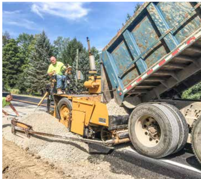
BERMING on Millsboro Rd. in Mansfield is Elite Excavating.
