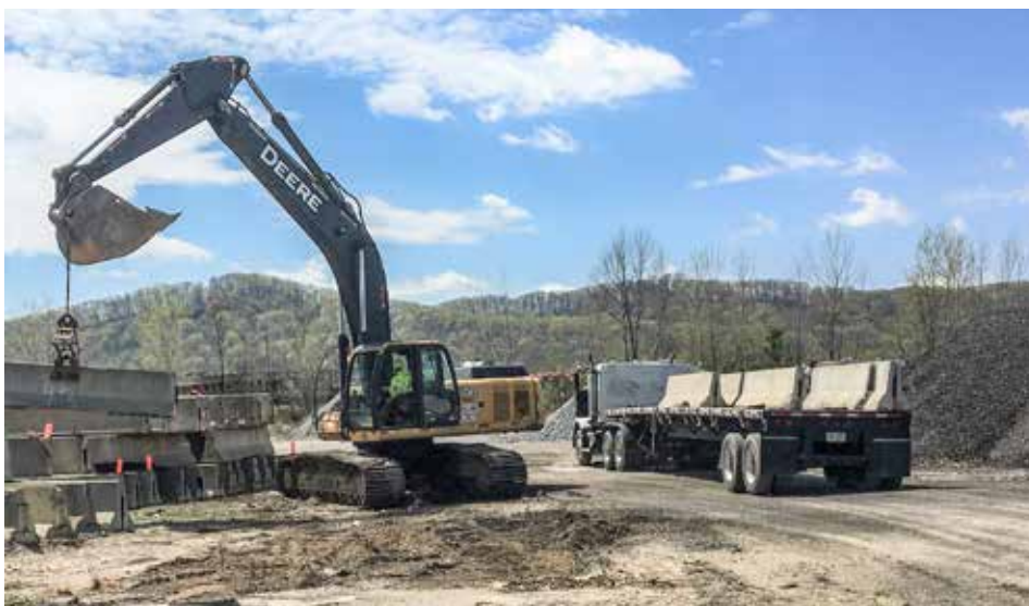
LOADING barrier wall for S.R. 207 at Higby Rd. in Ross County, Chillicothe is Mark Secrest, working for Shelly & Sands.
