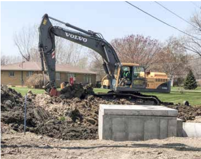
REPLACING a culvert on Barrett Rd. in Sandusky for Great Lakes Demolition is Tim Dearth.
