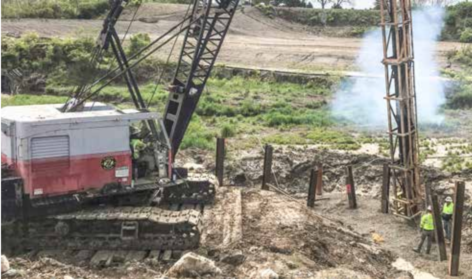
DRIVING piling at Marble Cliff for a pedestrian bridge in Franklin County is Double Z Construction.
