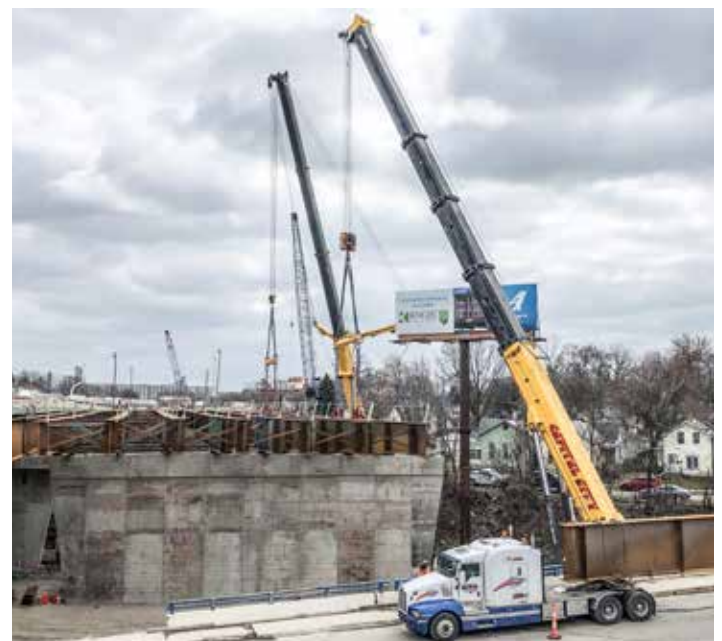
SETTING bridge beams on I-75 in Toledo is Capital City Crane.
