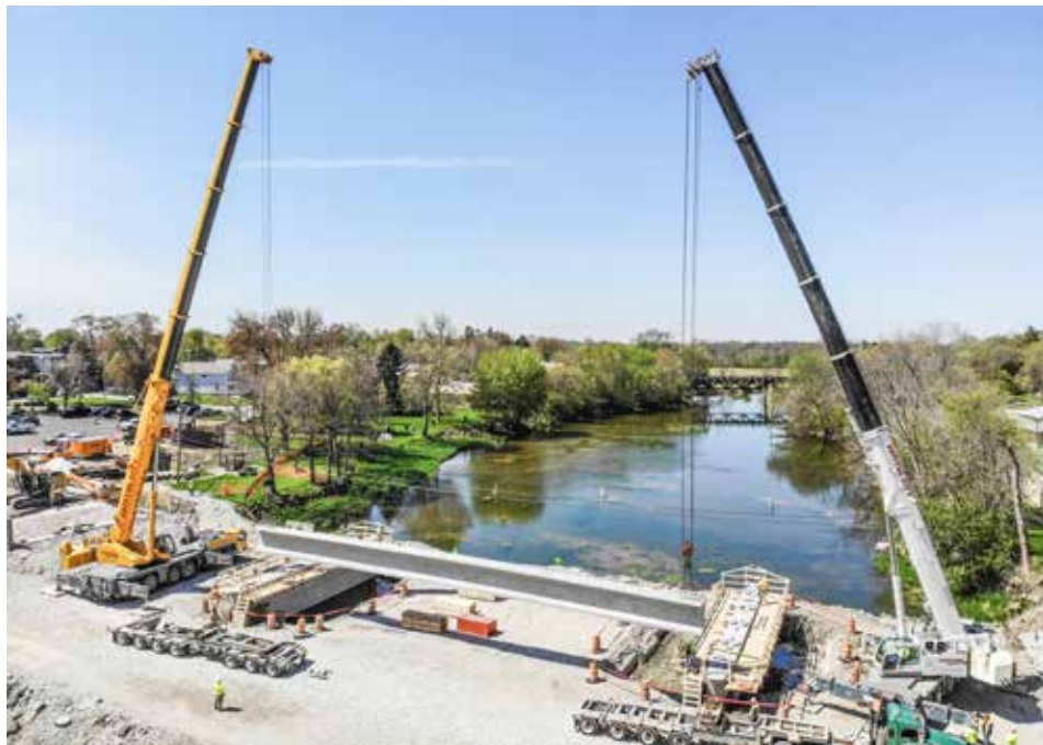
SETTING prestressed concrete bridge beams on Kokosing's S.R. 51 bridge over the Portage River in Elmore is Capital City.
