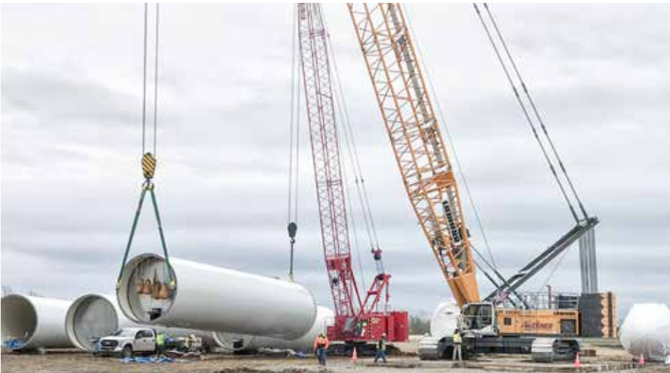
"TRIPPING" the base section on a turbine on the Scioto Ridge Wind Farm in Hardin County is White Construction.
