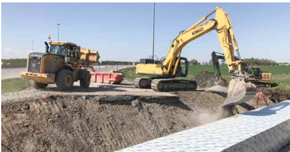
BACKFILLING an 84-inch box culvert in Beaverdam for Shelly are Jason Cline in the loader, Steve Harpest in the center backhoe and Dave M. Cross in the far-right excavator.
