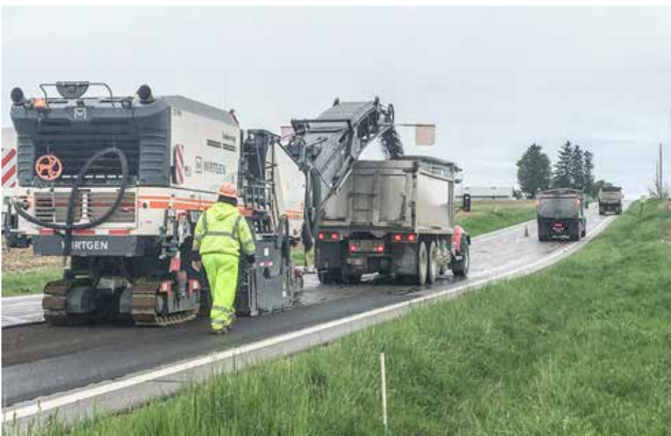
GRINDING on S.R. 3 in Wooster by Kokosing.
