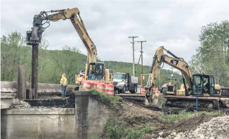
BUSY for Complete General at Otway Village in Scioto County on S.R. 73 are (l-r) Jason Forquer in the excavator placing sheet piling and Jasper Jenkins running an excavator.
