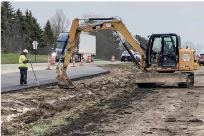
SLOPING ditches for Shelly & Sands on the turn lane project on U.S. Rt. 224 in Westfield Center is Carlos Gonzalez.
