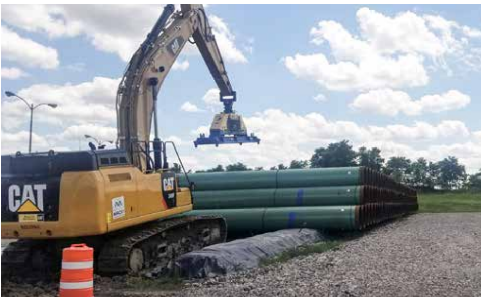
STRINGING pipe on the Buckeye XPress Pipeline in Rio Grande, Ohio is Mackie Logging.
