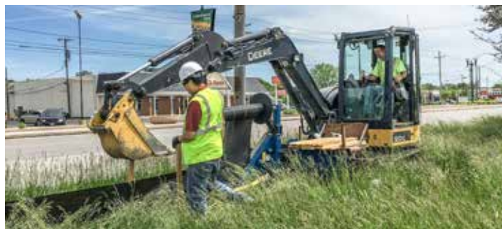
INSTALLING silt fence with an excavator at the new Amazon Distribution Center in Toledo is Victor Niese.
