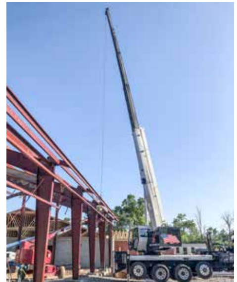
SETTING structural steel for a new fire station on Douglas St. in Vermilion for Gurtzweiler is Kirk Shank.
