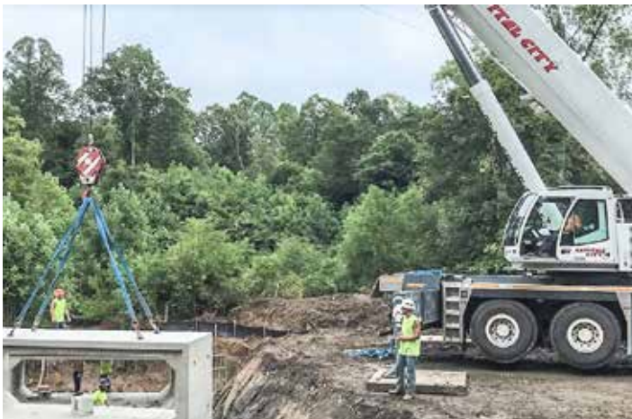
SETTING box culverts for Capital City Crane and Bud Inc. in Athens County is Brook McCune.
