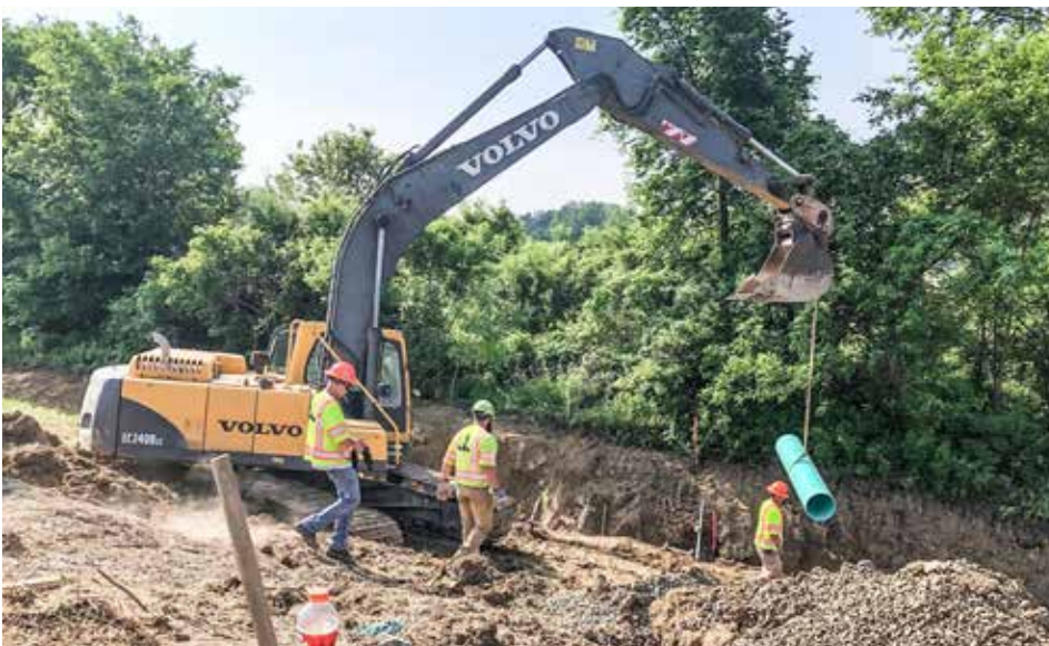
INSTALLING a storm sewer on the Ohio Turnpike in Milan for Gerken Asphalt is life member Martin Niese, operating an excavator.
