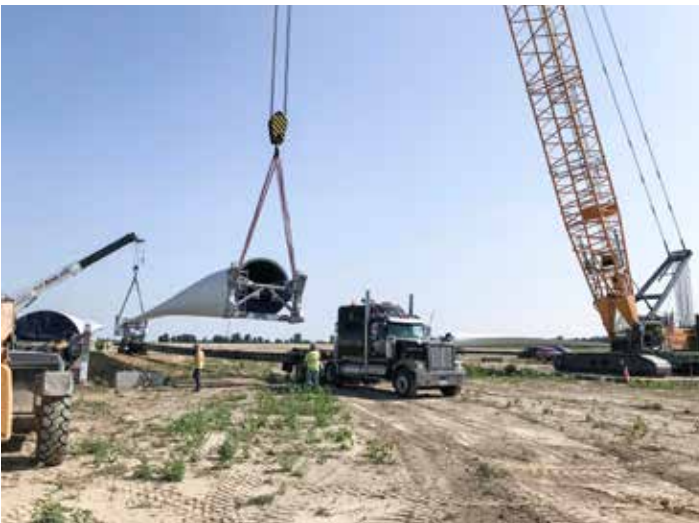
OFFLOADING blades on the Scioto Ridge Wind Farm in Hardin County is White Construction.
