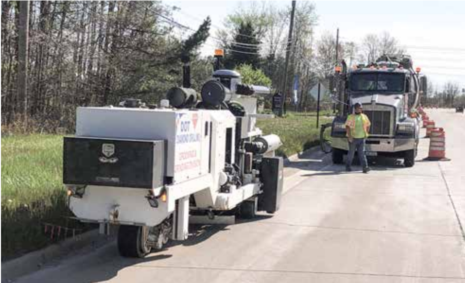
GRINDING Colorado Ave. in Sheffield for DOT Diamond Core Drilling are Bob Bentley, operating the diamond grinder, and Michael Gilreath, running the water truck.
