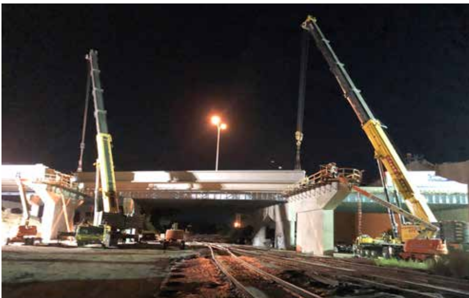
SETTING bridge beams on the I-75 reconstruction project in Toledo is Capital City Crane.
