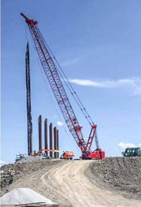
DRIVING piling for Flatiron Bridge Project in Brilliant, Jefferson County.
