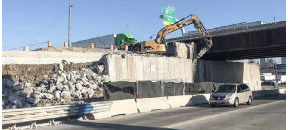
HAMMERING a bridge abutment on I-75 in Toledo for E.S. Wagner is Alexandyr Scholl.
