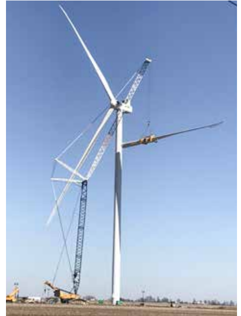
"STABBING" a blade with a Liebherr 1750 on the Timber Road IV Wind Farm in Paulding County is Kiewit Power Constructors.
