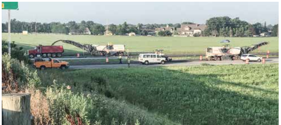
MILLING project on U.S. Rt. 20 in Fremont, Ohio by Ebony Construction.
