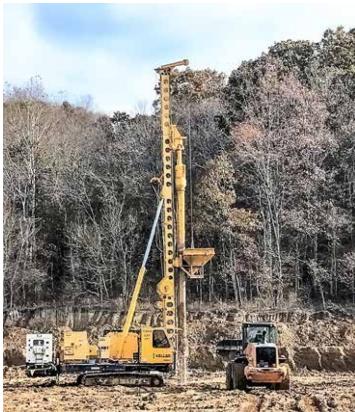
PUTTING in geo piers in Logan, Hocking County is Hayward Baker.
