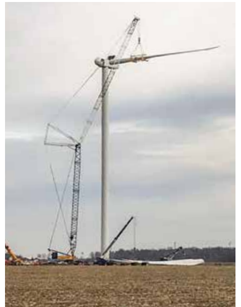
"STABBING" a blade utilizing a Liebherr 1750 on the Timber Road IV Wind Farm in Paulding County is Kiewit Power Constructors.
