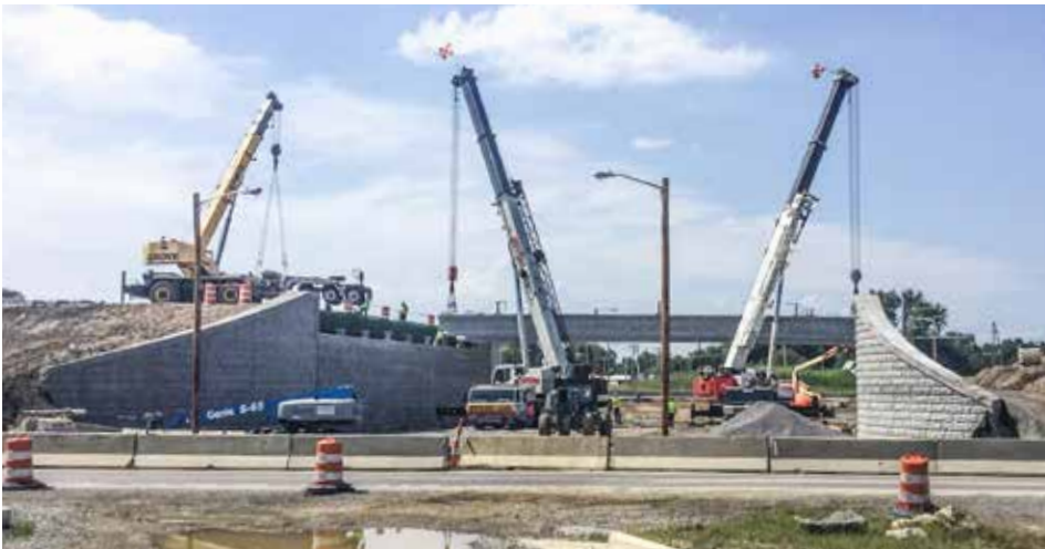
SETTING bridge beams on I-75 over Lima Ave. for Beaver Excavating in Findlay is Jeffers Crane Service.
