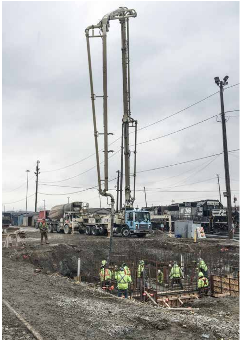
PUMPING concrete for a new fuel station at the Norfolk Southern Railroad yard in Bellevue for Howard Concrete is Ed Vanko.
