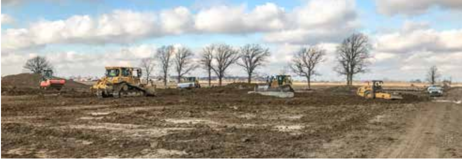
BACKFILLING a turbine base on the Scioto Ridge Windfarm in Hardin County is White Construction.
