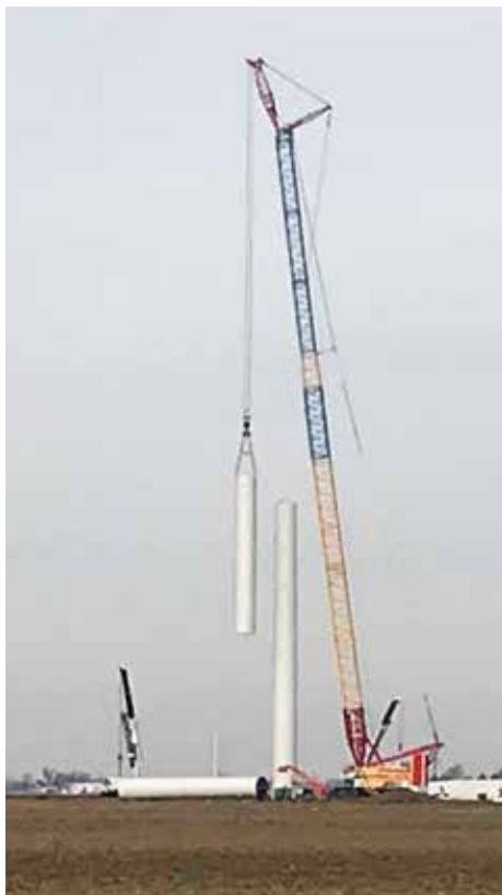
SETTING a "can" with a Liebherr 11000 on the Timber Road IV Wind Farm Project in Paulding County is Kiewit Power Constructors.
