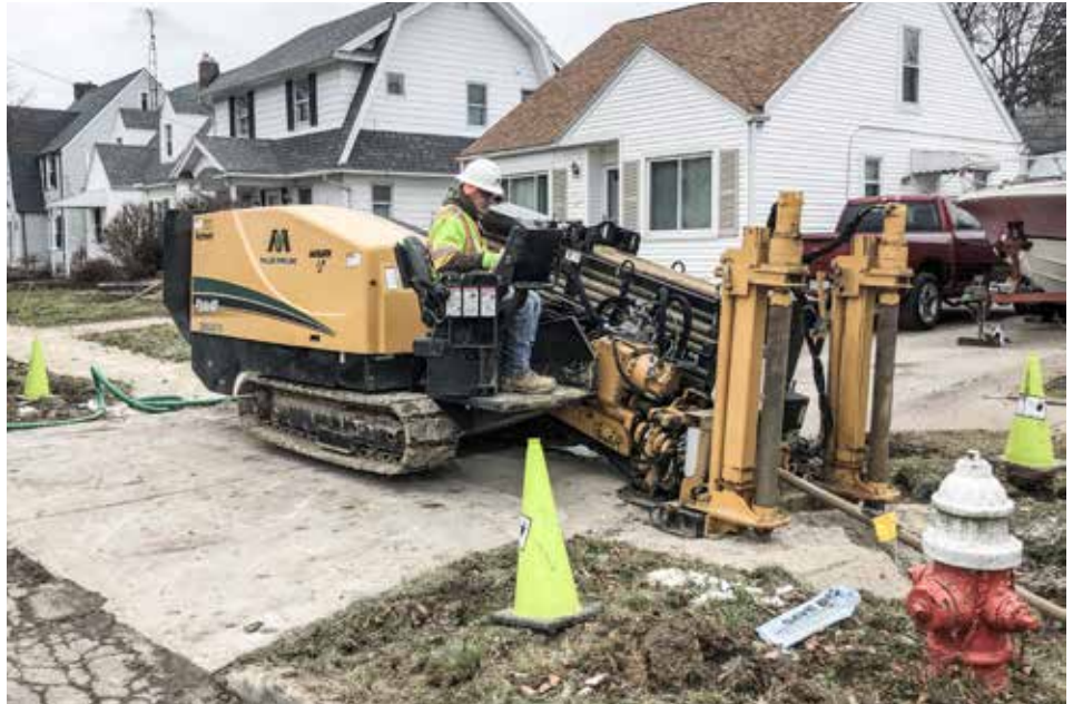
REPLACING gas line in Point Place for Miller Pipeline is Harper Harris.
