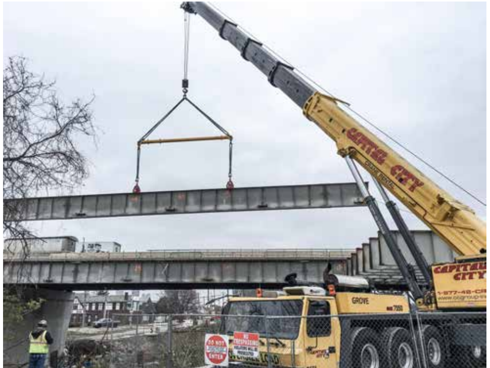
PULLING beams on I-75 in Toledo is Capital City Crane.
