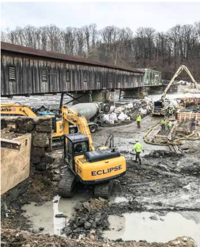
BUILDING a dam in Harpersfield is ECLIPSE, with Howard Concrete pumping the concrete.
