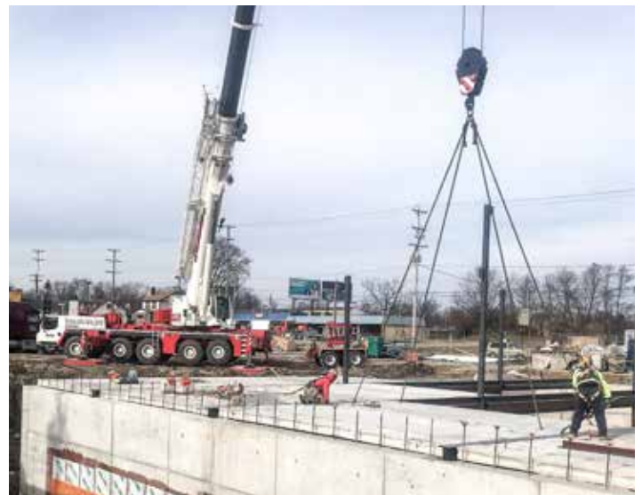
SETTING hollow-core decking at a new fire station in Columbus is ALL Crane of Columbus.
