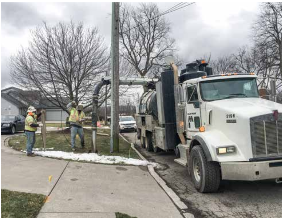
ON THE JOB hydro-excavating for Miller Pipeline in Point Place are (l-r) Matthew Mellot and Levi Crooks.
