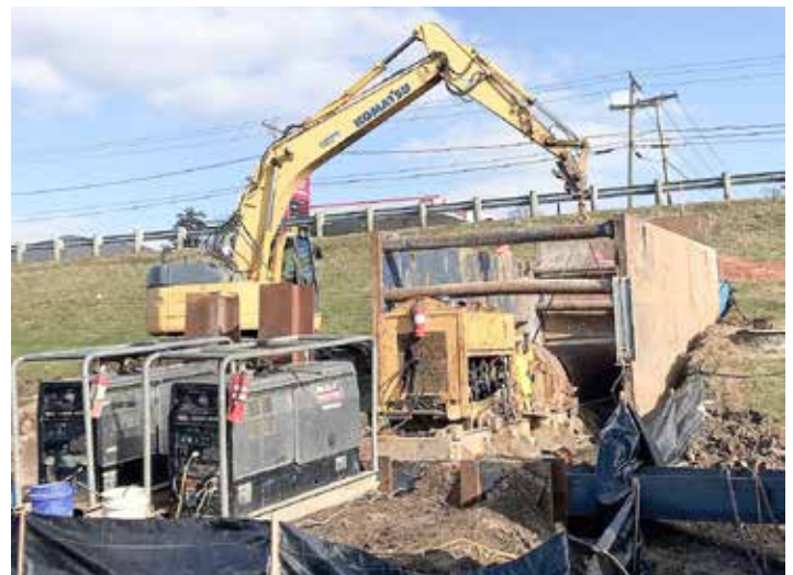
BORING under Memorial Drive in Lancaster, Fairfield County is Capital Tunneling.
