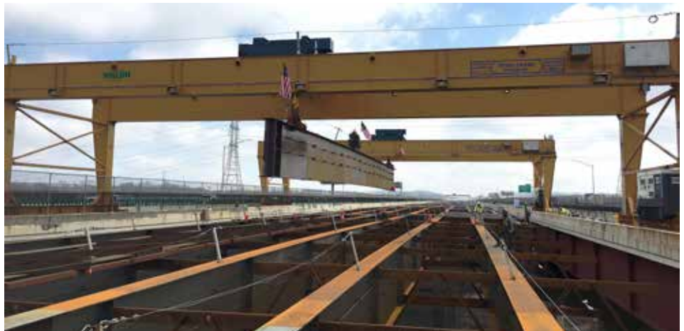
INSTALLING the final beam on the I-480 Union Workers Memorial Bridge.
