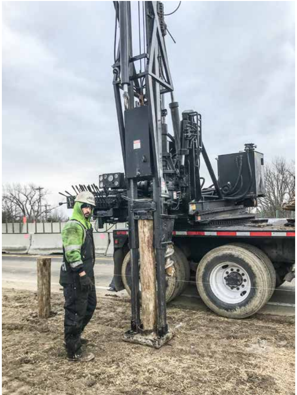
OPERATING a post-pounder for Security Fence in Clark County is Deontre Borgman.
