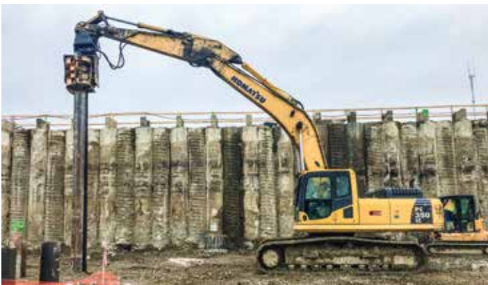
DRIVING piling for George J. Igel & Company at Crew Stadium in Columbus, Franklin County is John Raines.
