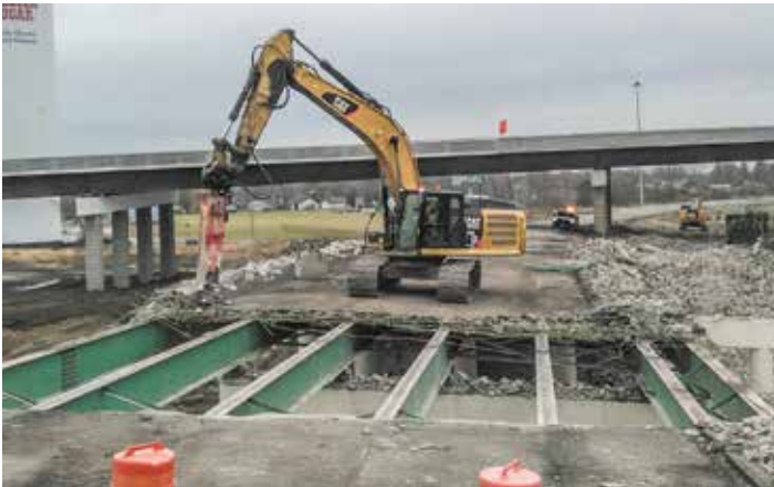
DEMOLISHING a bridge deck on I-75 in Findlay is Beaver Excavating.
