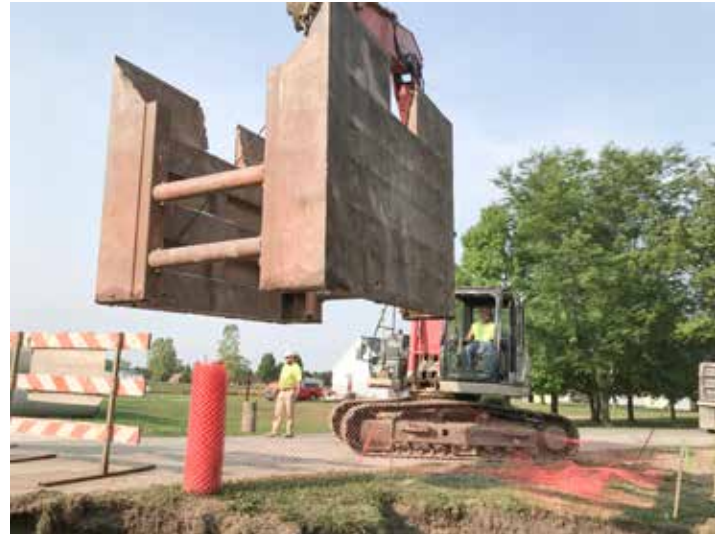
SETTING a trench box for B. Hill's in Vanlue is Matt Sheets.
