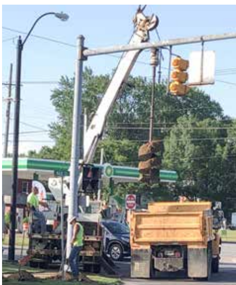
DRILLING traffic light foundations on Main St. in Huron for Miller Cable is Dana Dickman operating a digger derrick.
