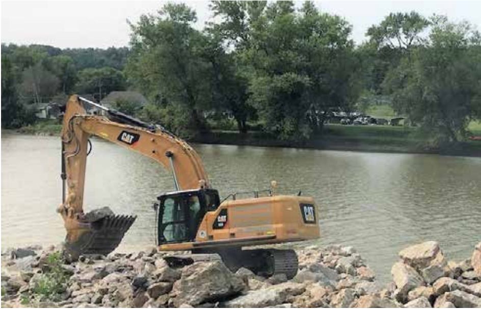
PLACING rip rap on a slide repair on S.R. 60 on the Muskingum River in Morgan County is Beaver Excavating.
