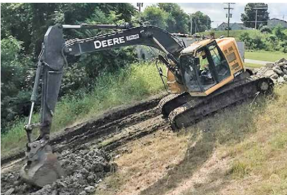
BUSY at Duncal Falls placing rip rap for Complete General in Muskingum County is Tim Waites.
