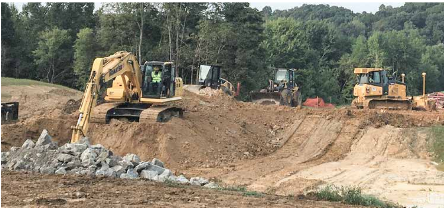
INSTALLING a new spillway and repairing overflow for Beaver Excavating on Tycoon Lake in Gallia County are Calvin Jordan on the excavator and Garret Kaldor on the dozer.
