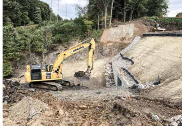
REPAIRING a slip and extending a culvert on Dean Rd. in Birmingham for Great Lakes Construction are Jim McClafin running the Komatsu hoe and life member Doug Bowman running the compactor.
