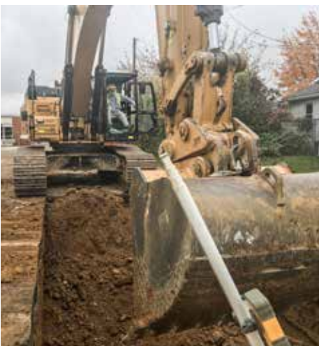
INSTALLING pipe at the new Lexington High School is Beaver Excavating.
