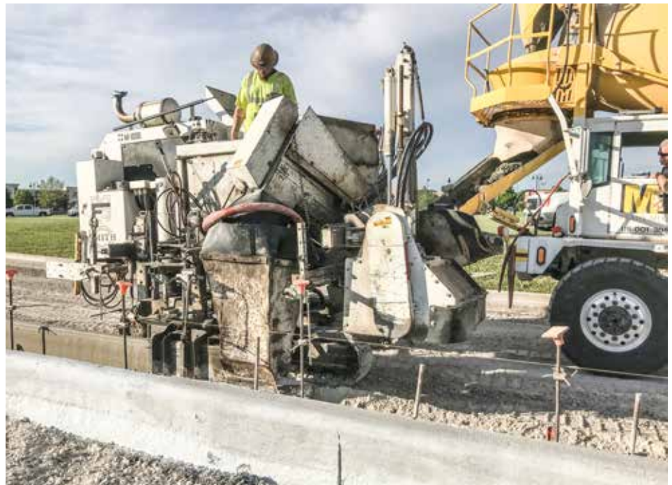
INSTALLING curb for Smith Paving at the Amazon project in Rossford is David Brown, Jr.
