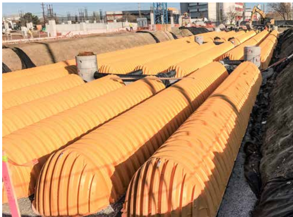
INSTALLING an underground storm water detention system at OSU, Franklin County is McDaniels Construction.
