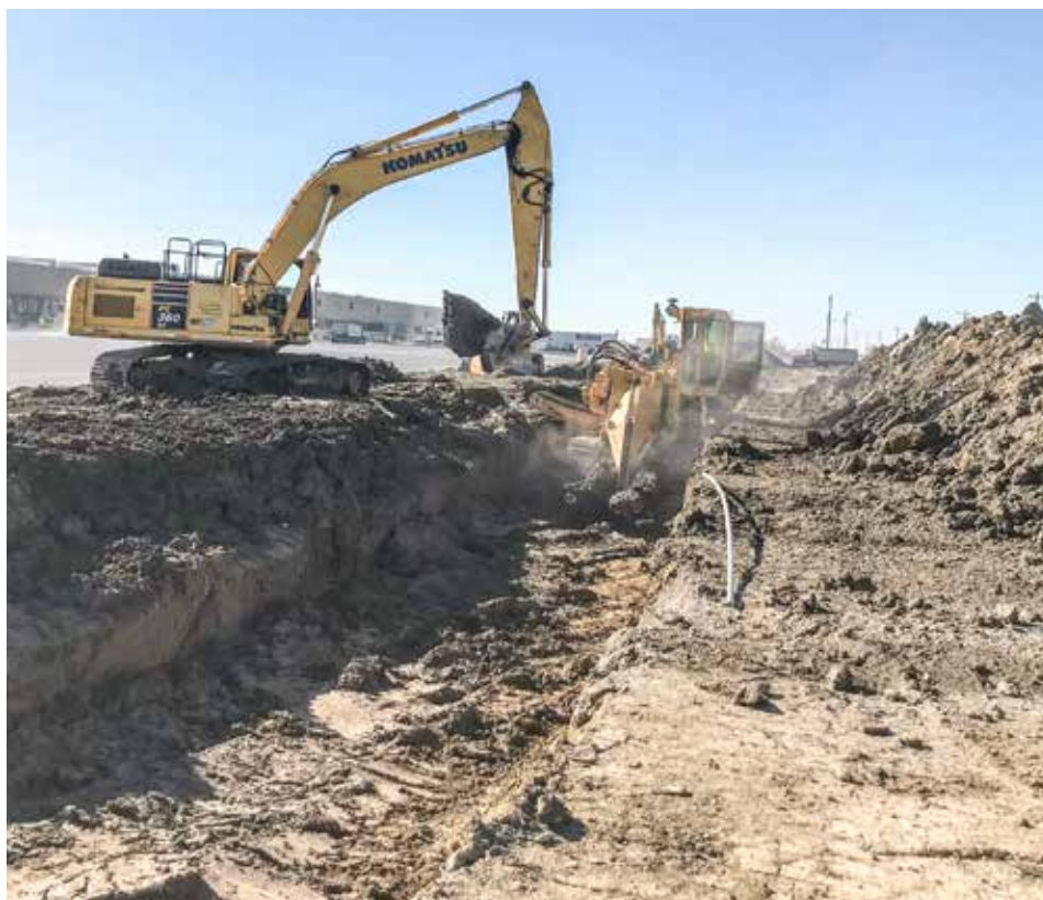
CUTTING a 24-foot deep trench in preparation for a sewer line in North Baltimore is Underground Utilities.
