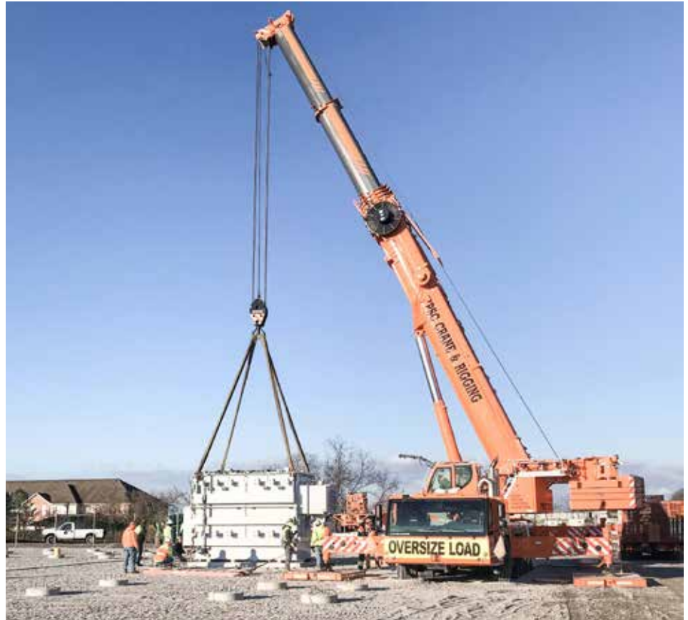
SETTING a transformer at the new Hamilton substation on a Great Lakes Construction project for Piqua Steel Company is R. Tyler Sanderson.
