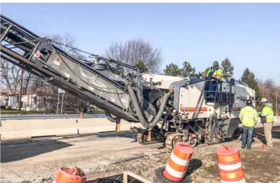
OPERATING an asphalt mill on the Anthony Wayne Trail in Toledo is Shannon Scott.
