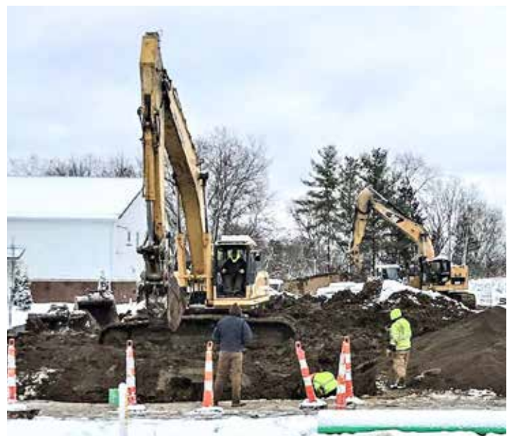
INSTALLING new sanitary sewer in Granville, Licking County is Elite Excavating.
