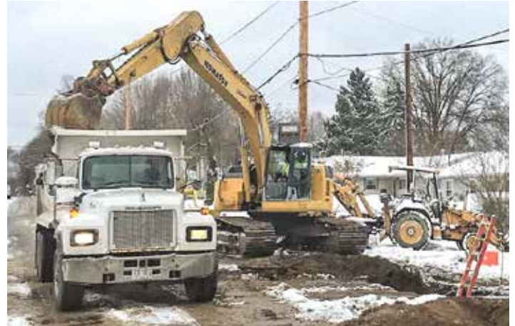
INSTALLING new water main in Newark on 40th St., Licking County is Fabrizi Trucking.
