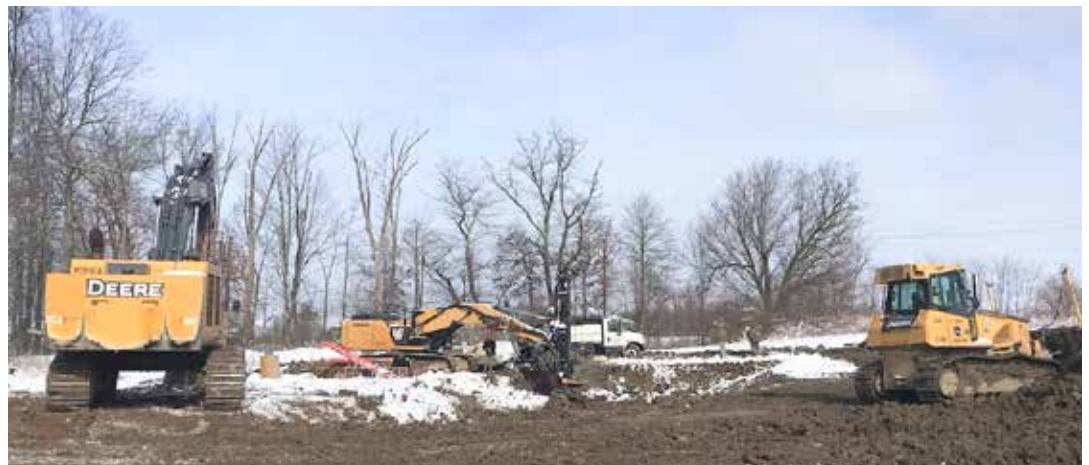
PUTTING in a drill pit to tunnel under S.R. 161 in New Albany, Franklin County is Complete General.
