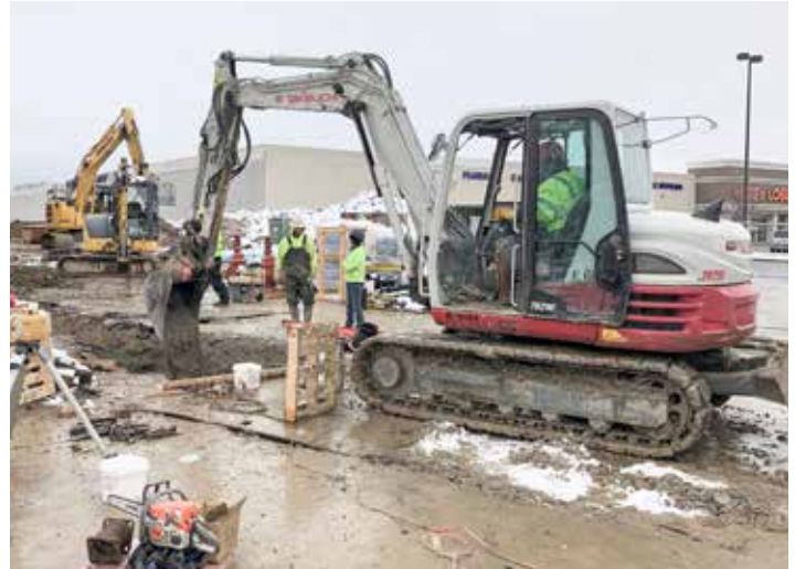
DIGGING a fire line at the Sandusky Mall for Fabrizi are Russel Fitch and Victor Garcia. Russel is operating the Takeuchi hoe and Victor is operating the Komatsu hoe in the background.
