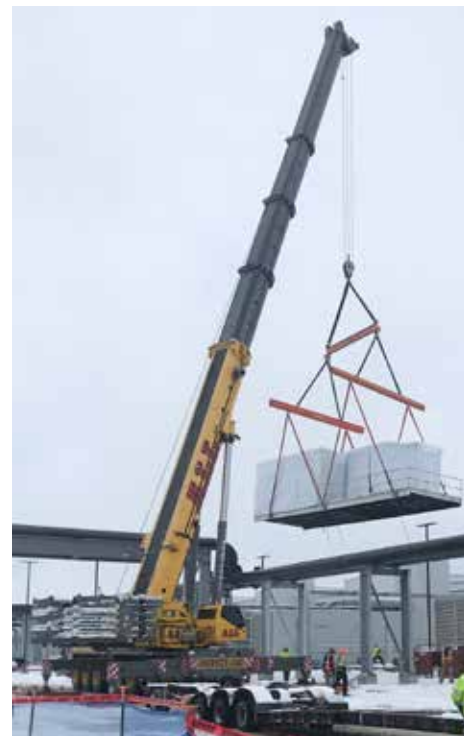
SETTING mechanical systems at Mustang in New Albany, Franklin County is ALL Crane.
