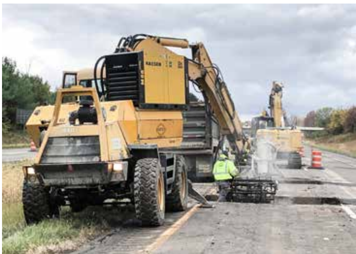
WORKING for Smith Paving on the U.S. Rt. 20 bypass in Norwalk are Dustin Hermes and Sean McFadden. Dustin is drilling dowels with the Badger rubber tire hoe and Sean is in the Kobelco hoe digging out the repair patches.
