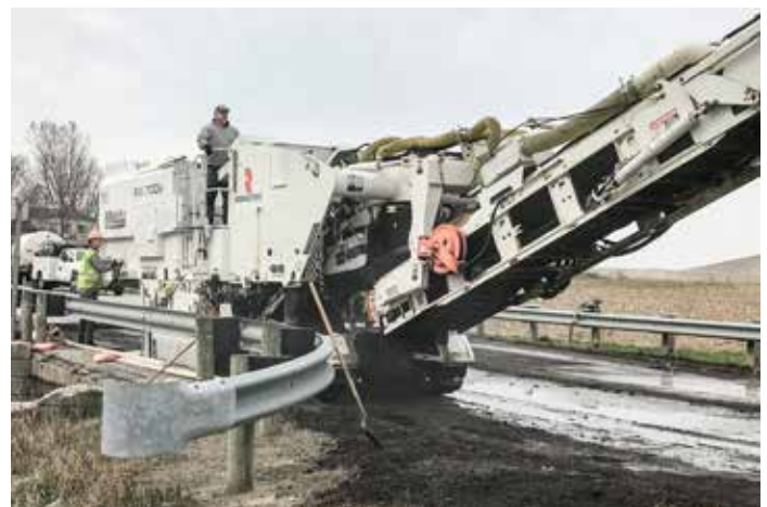
MILLING asphalt on U.S. Rt. 23 in Seneca County, south of Fostoria, for Welfle is Raul Hinojosa.
