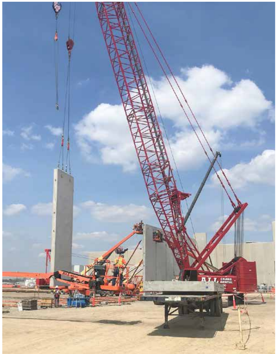
SETTING precast walls at Project Mustang in New Albany, Franklin County is ALL Crane.
