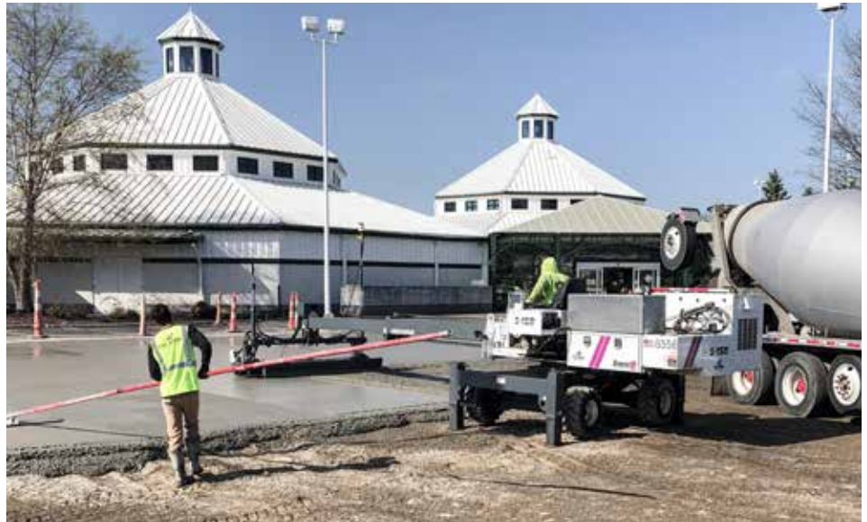
OPERATING the power screed for Tri Mor at Petitti's in Avon is Brandon Mandich.
