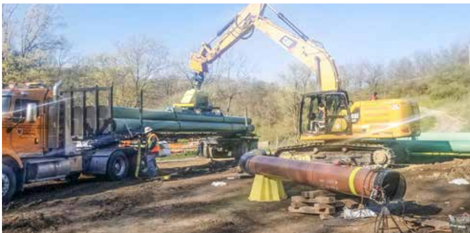
WORKING on a 20" new lay for Antero in Monroe County is Integrity Kokosing Pipeline Services.
