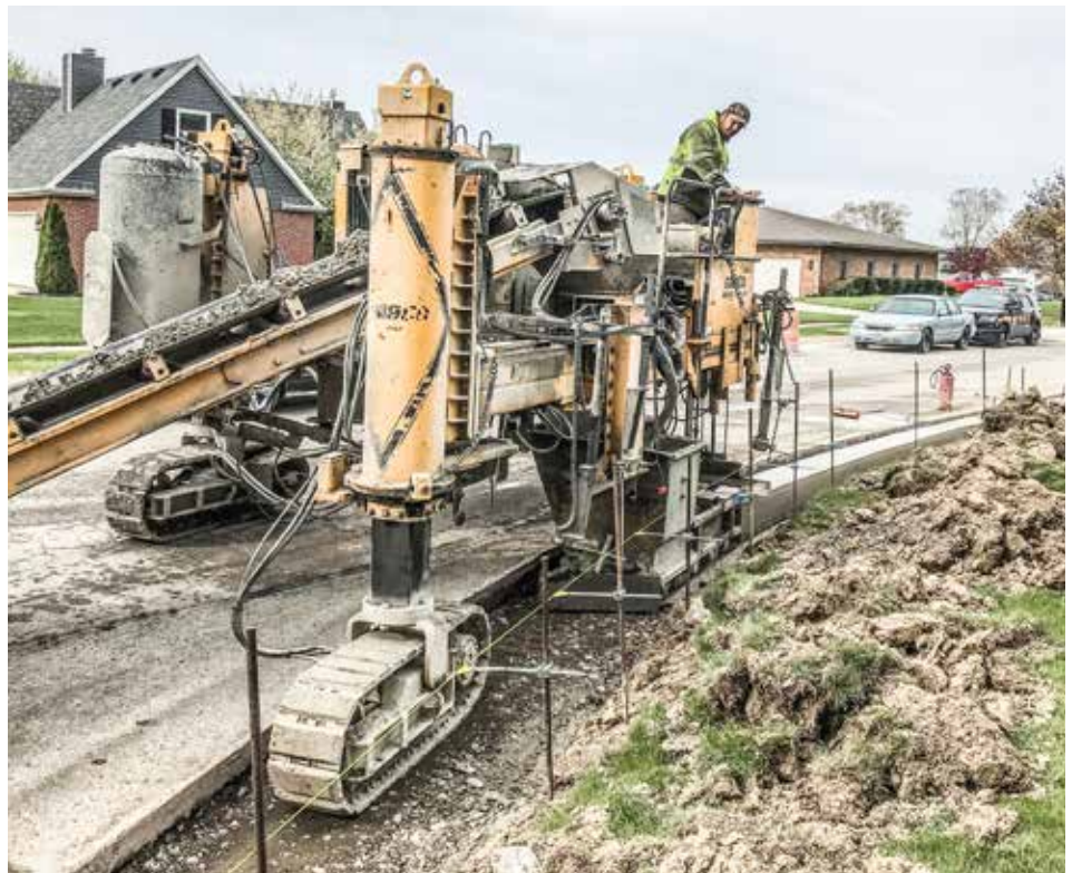
SLIPPING curb & gutter on Foxbury Lane in Findlay for Smith Paving is Dave Brown.
