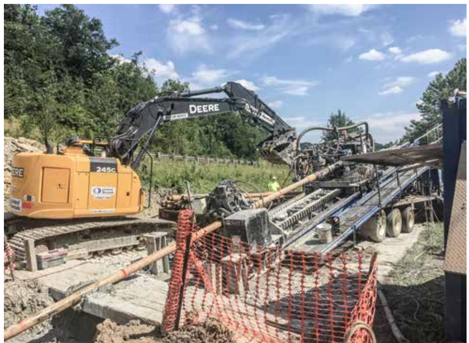
HDD DRILLING in Northern Kentucky is Aaron Enterprises.
