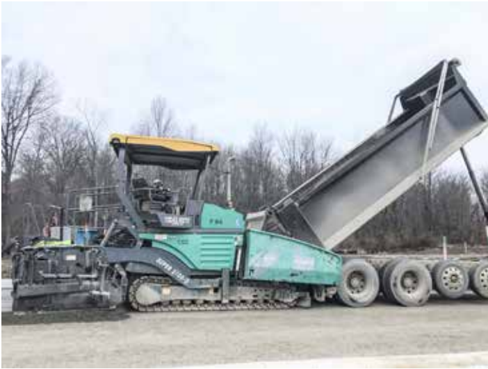
PLACING RCC in Pataskala, Licking County is Complete General.
