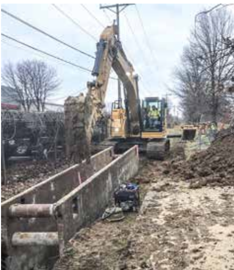
INSTALLING ductile iron pipe for a sludge line for the City of Columbus on Morse Rd., Franklin County is Complete General.
