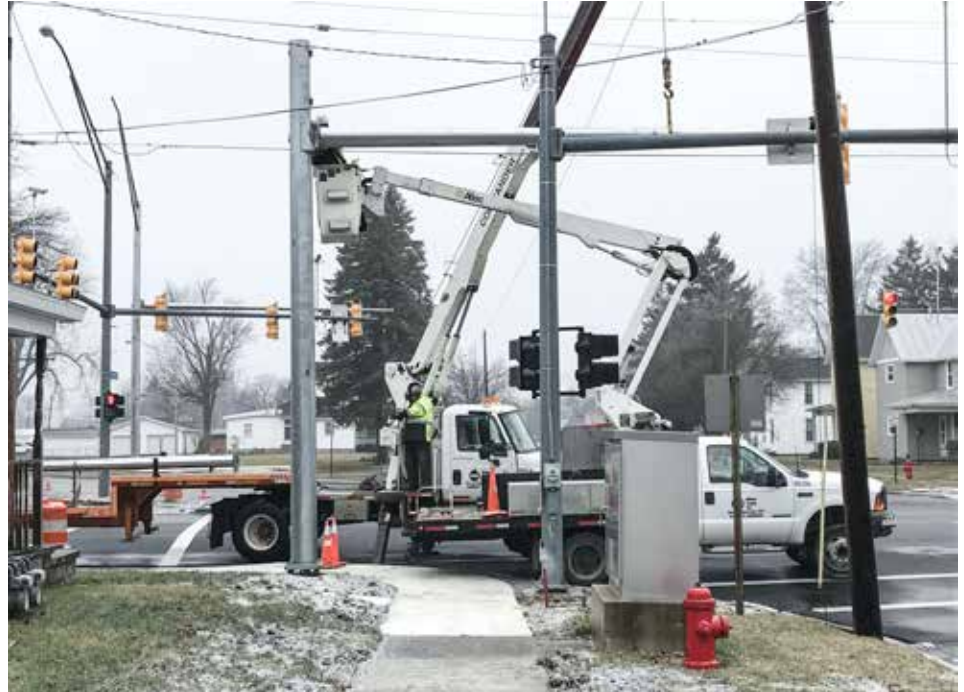
REPLACING traffic signals on Blanchard St. in Findlay for Miller Cable is Chad Whitman.
