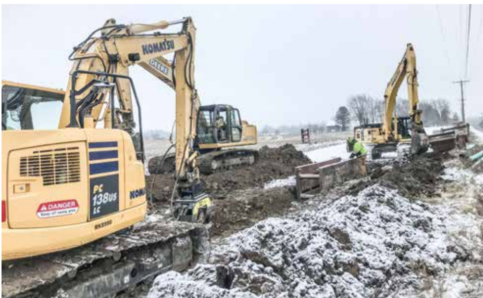
LAYING sanitary sewer line in Russia is Kinnison Excavating.
