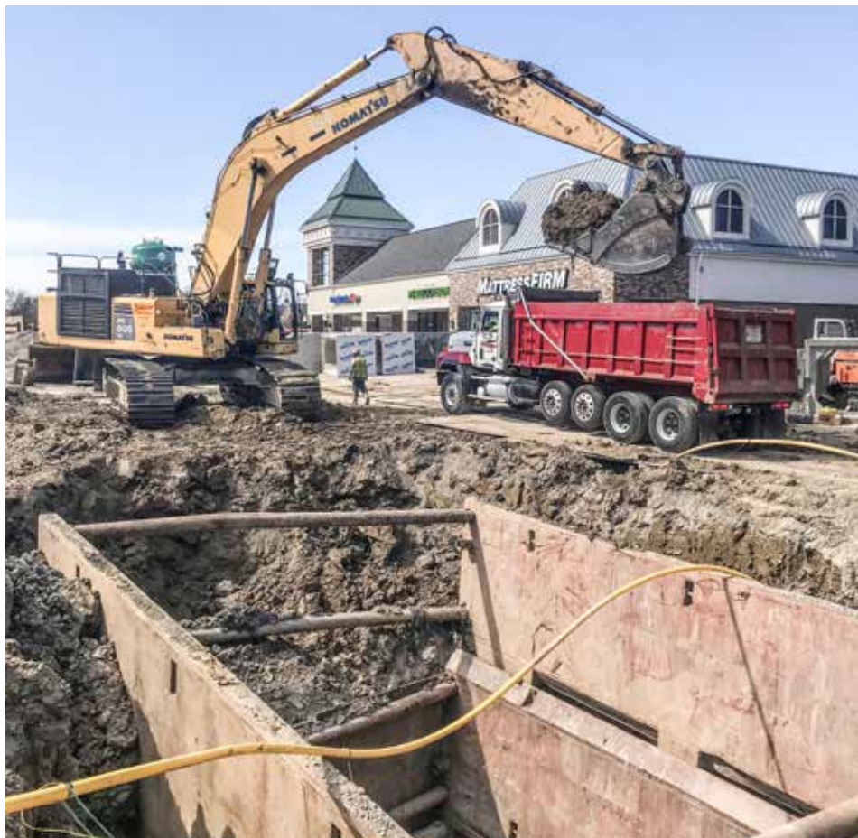
DIGGING a 34-ft. deep sewer in Strongsville for Fabrizi Trucking & Paving is operator Mark DeAnna and oiler Brian Otto.
