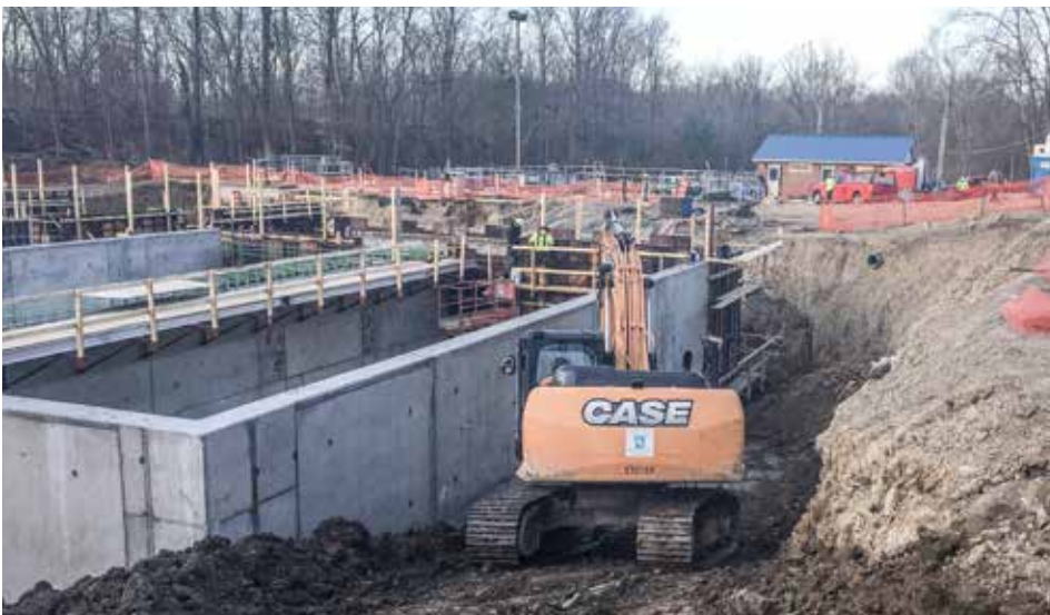
BACKFILLING at the West Salem Wastewater Treatment Plant for Stanley Miller is Ronald "Jeff" Holland.
