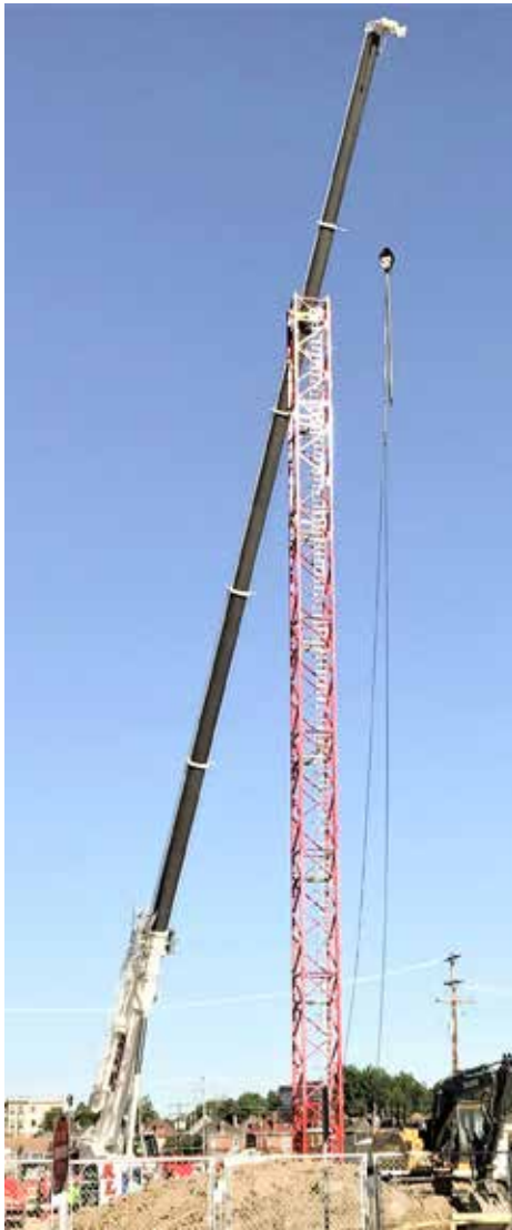
ERECTING a tower crane in East Columbus, Franklin County is ALL Crane.
