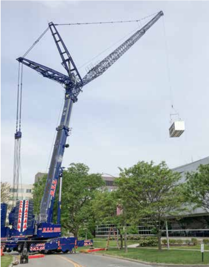
SETTING new air units for the VA Hospital in Cleveland using a 770-ton Liebherr with 285-foot of jib for ALL Crane is operator John Belu.
