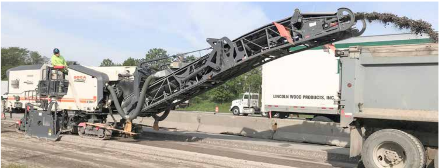
MILLING asphalt for Shelly & Sands on I-71 in Columbus, Franklin County is BOCA.
