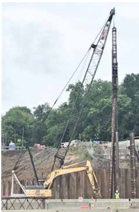
DRIVING piling for bridge replacement in Granville on S.R. 37, Franklin County is Shelly & Sands.
