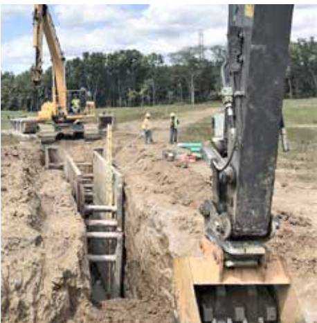
INSTALLING sanitary sewer in Grove City, Franklin County is Trucco Construction.
