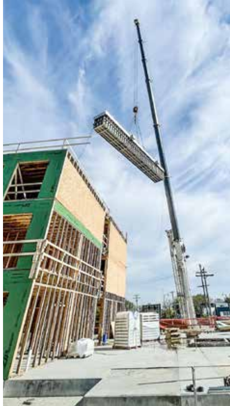
SETTING a pool for the Waterford Bluffs at W. 20th and Lorain Rd. in Cleveland is General Crane.
