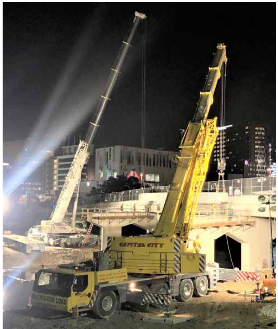
SETTING bridge beams for Kokosing at OSU, Franklin County is Capital City Group.
