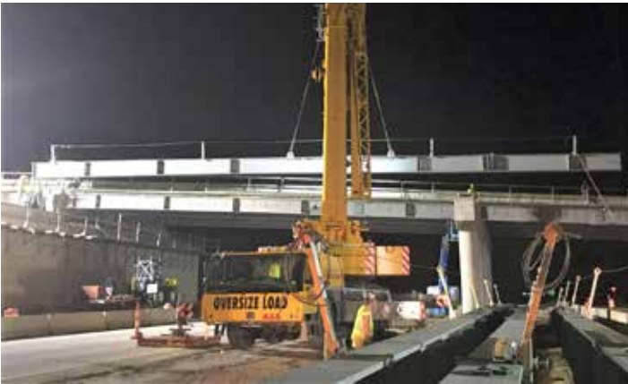
SETTING bridge beams for Shelly & Sands on S.R. 37 is Capital City Group.
