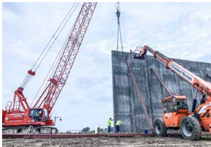
TILTING up walls at the First Solar facility in Perrysburg is Capital City Crane Rental.
