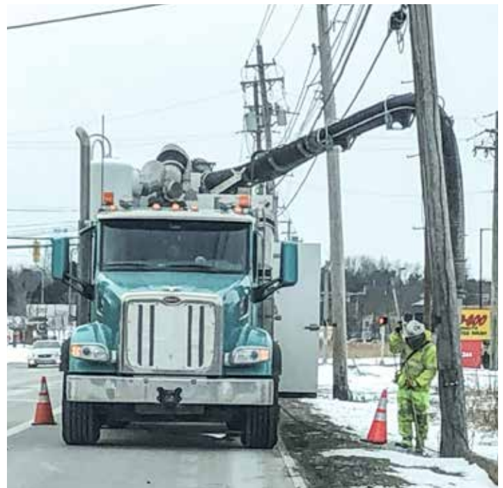
HYDRO excavating telephone pole holes on Center Rd. in Avon for Badger Daylighting is Tom Seaman.
