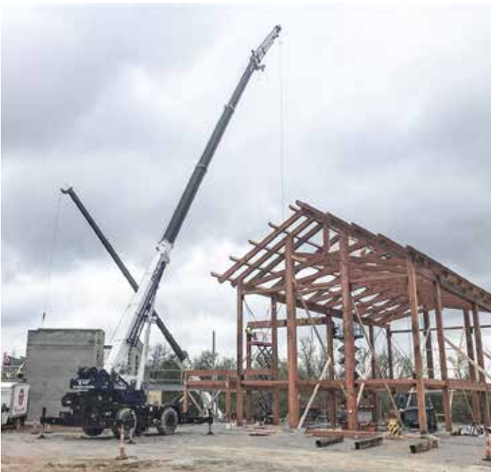
SETTING structural wood beams for PSC Crane & Rigging at the new lodge at Old Man's Cave, Hocking County is Brandon Cox.
