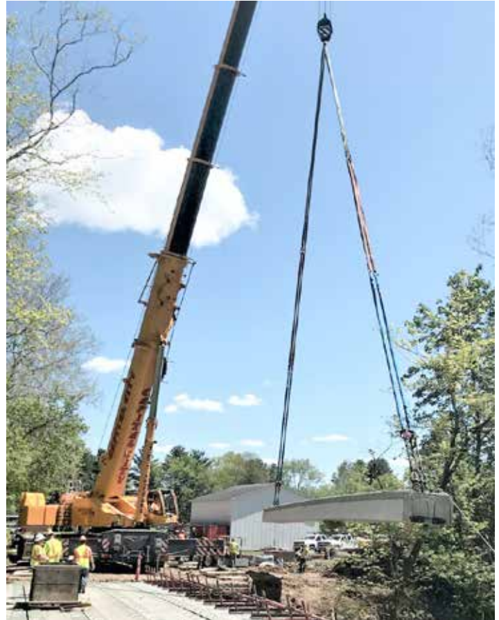
SETTING bridge beams for Axis Civil Construction on Woodlane Ave. in Nelsonville, Athens County is Capital City Crane.
