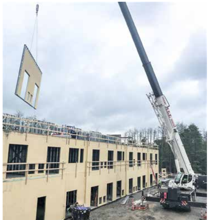
SETTING prefab wall panels at Old Man's Cave for the hotel portion of the new lodge in Hocking County is Joseph Hibbard.
