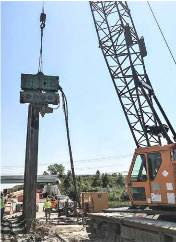
PULLING sheet piling for Kokosing on I-71 in Grove City, Franklin County is Douglas Crider.
