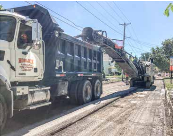
MILLING Church St. in Bowling Green is Morlock Asphalt.
