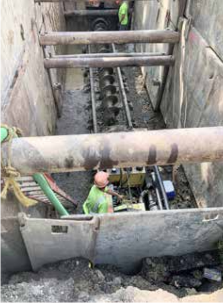
OPERATING a bore machine for Underground Utilities in Huron is Al Thayer.
