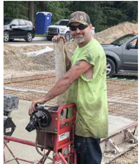
RUNNING a power screed for Karvo in Portage County is Tim Mihal.
