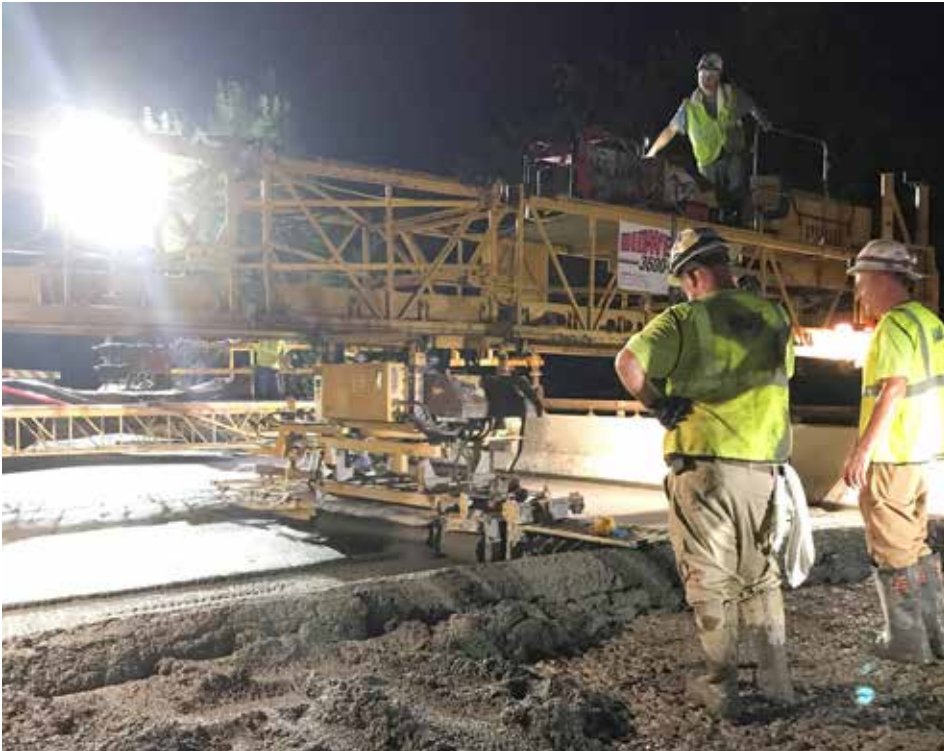
OPERATING a Bidwell on a new bridge deck over the CSX railroad for Great Lakes Construction on University Blvd. in Middletown is Lynn Ringenberg.
