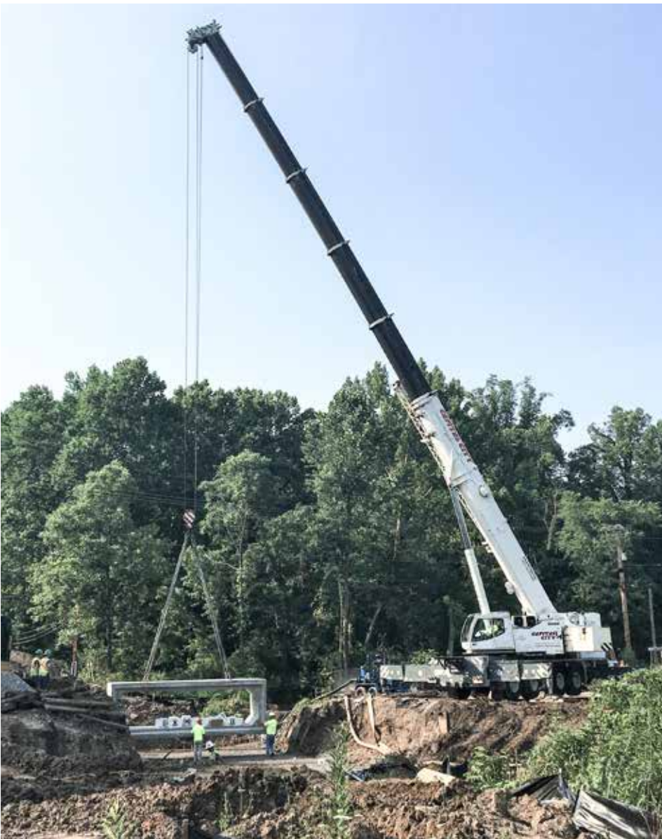
SETTING a box culvert in Lawrence County on C.R. 169 for Captial City Crane is Brian Norden.
