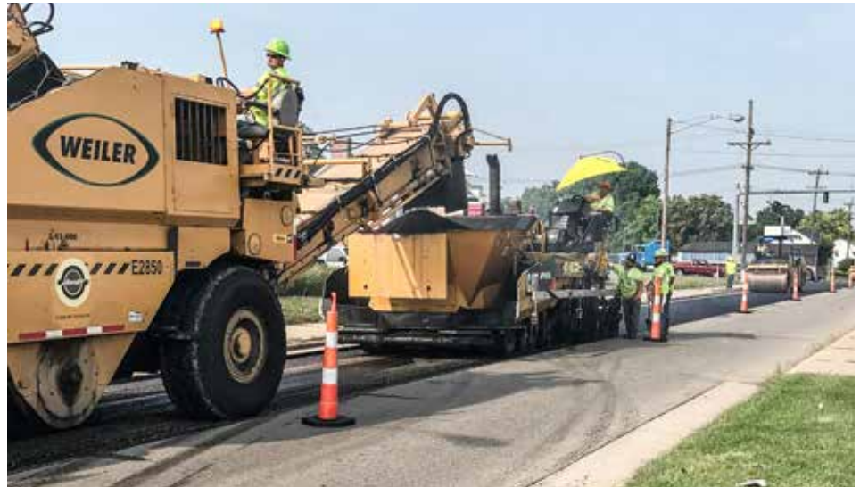
MILL and fill on S.R. 73 in Middletown on Verity Parkway by Barrett Paving. Brandon Ratliff is on the shuttle buggy, Scott Huxel and Larry Colley are on the rollers.
