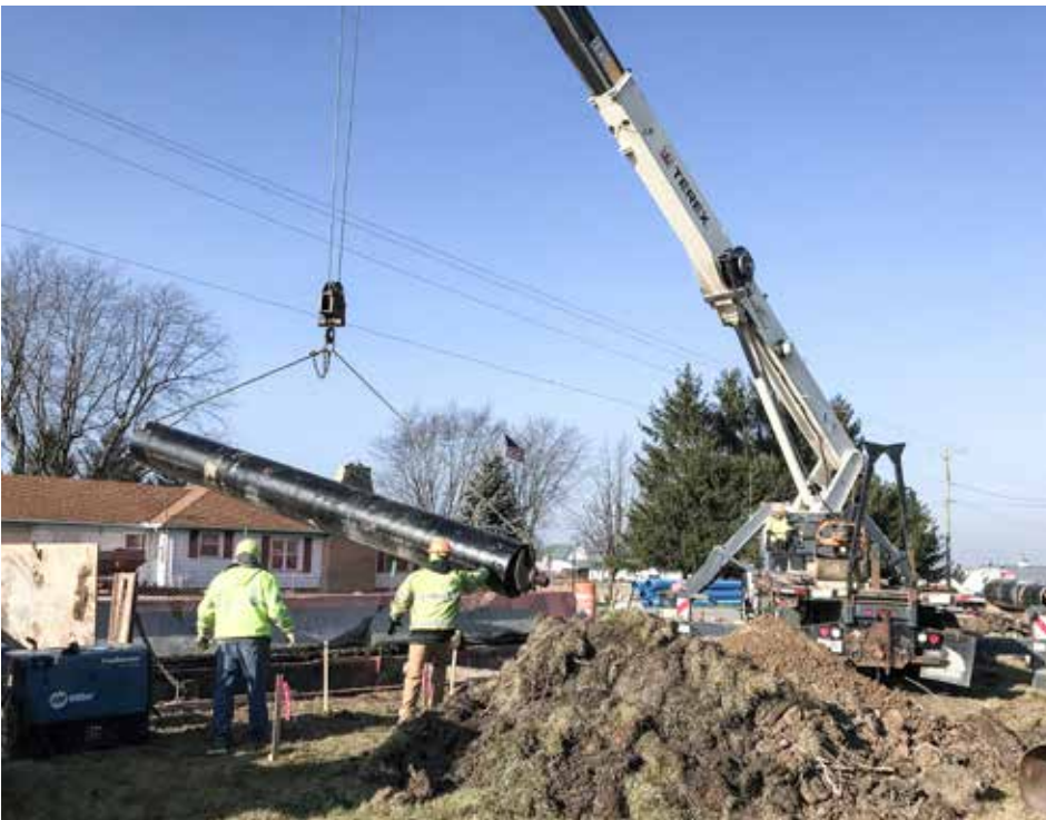
INSTALLING a new water line on Napoleon Rd. in Allen County for Underground Utilities is Scott Riley on the boom truck.
