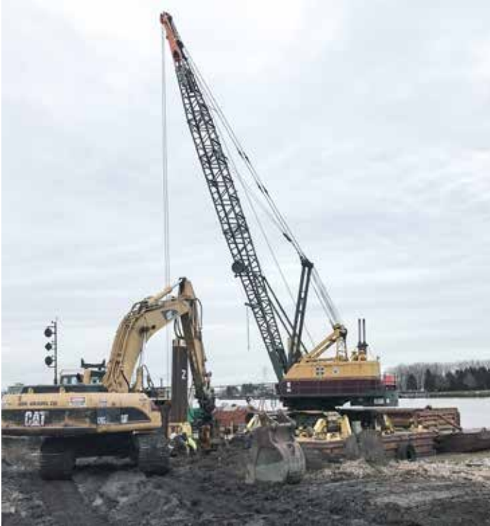
DRIVING sheet piling on the Maumee River in downtown Toledo is The George Gradel Company.
