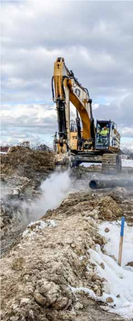
INSTALLING storm sewer in Aurora is Fechko.
