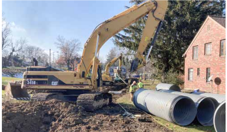
INSTALLING storm sewer in Mansfield is Underground Utilities.
