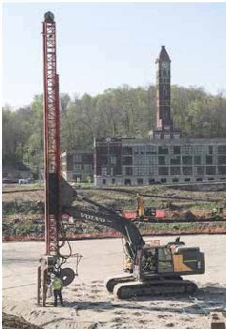
INSTALLING water wics for Eagle Bridge in Warren County is DGI Menard.
