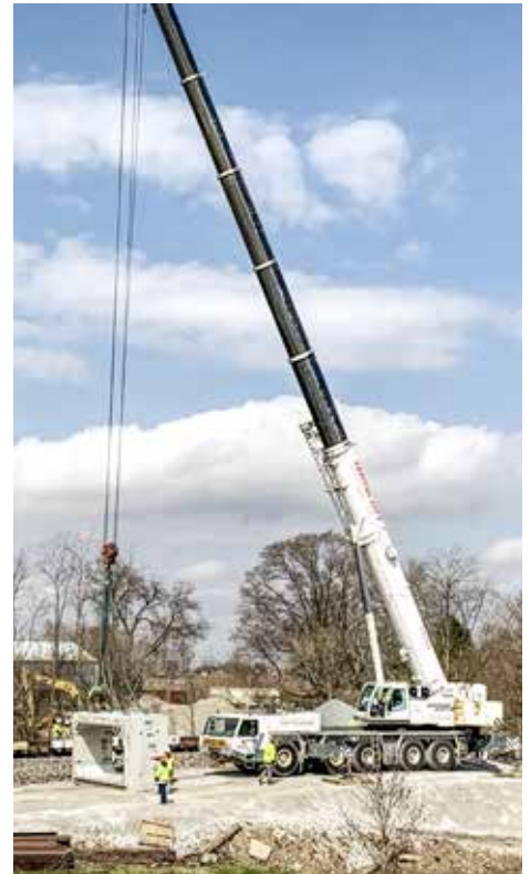
REPLACING a culvert in McComb is Capital City Crane.
