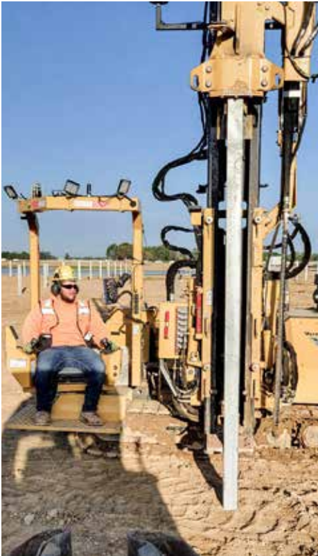
PERFORMING pile driving work for Kiewit on the Yellowbud Solar Project is Marcus Dille.
