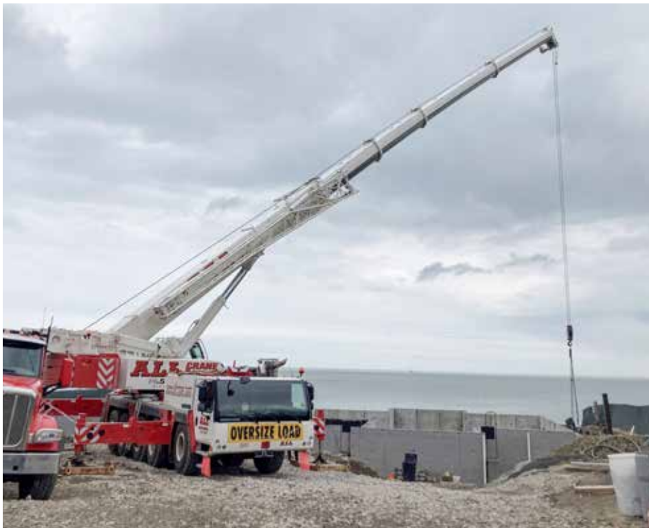
SETTING a residential precast wall on Harborview Ave. in Cleveland for ALL Crane is oiler Kane Capone and operator Mike Herbold.
