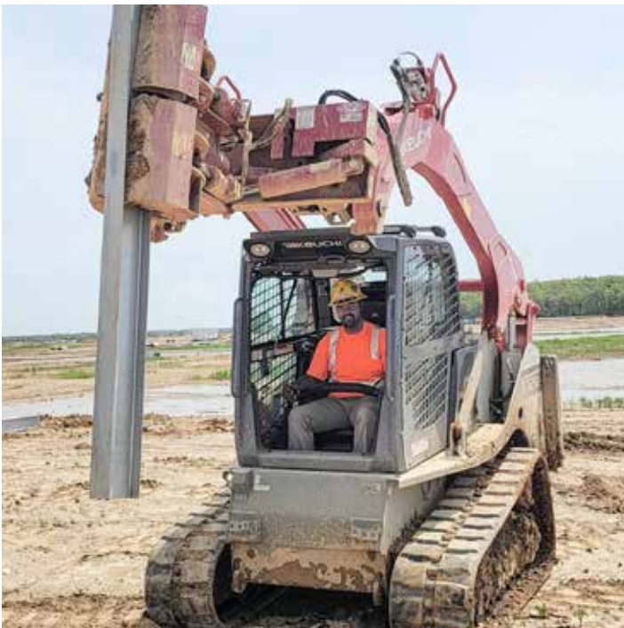
PERFORMING pile driving work for Kiewit on the Yellowbud Solar Project is Justin Lett.
